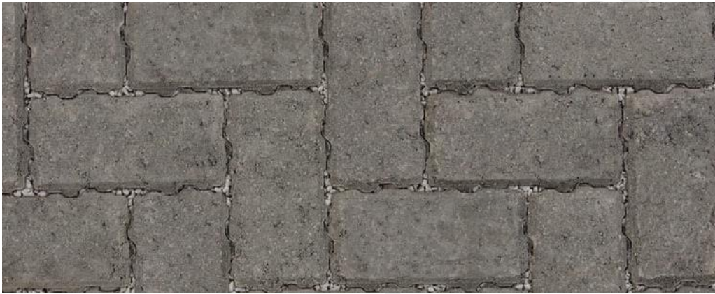
Block paving to front Marshall's Driveline Priora concrete block paving colour Charcoal.
