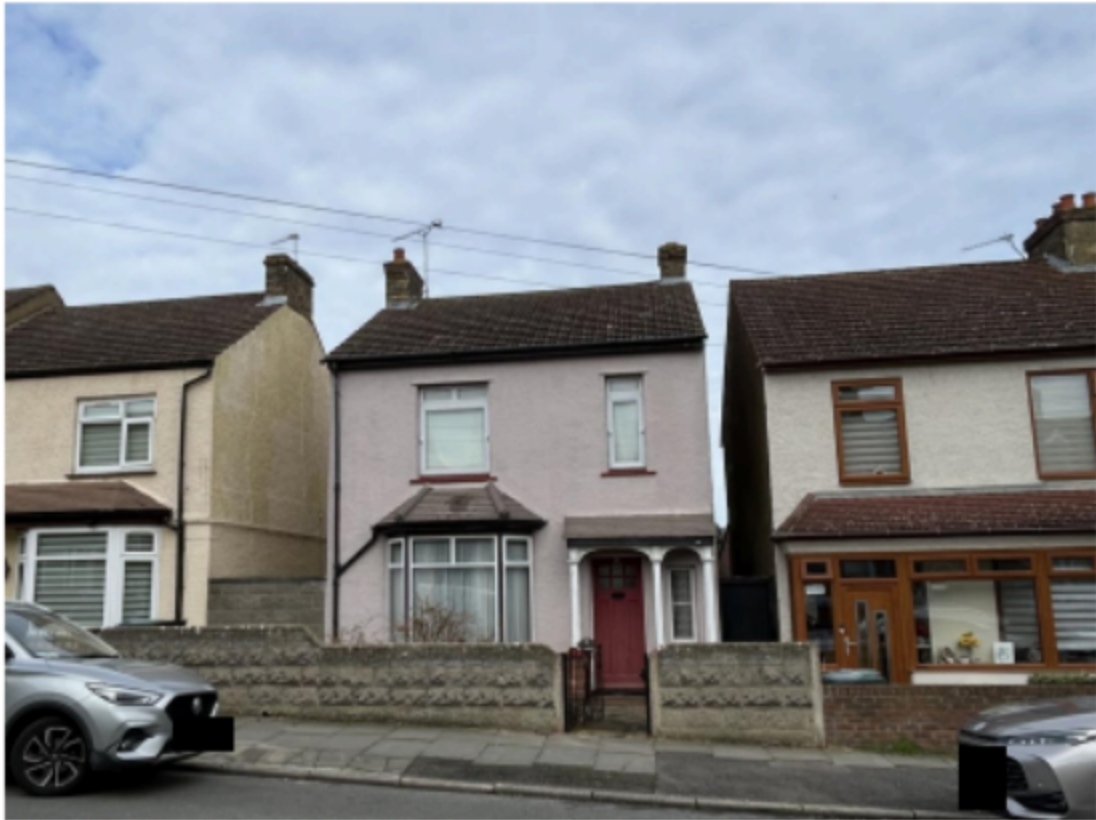
Photo 1. Front View – Park Avenue
