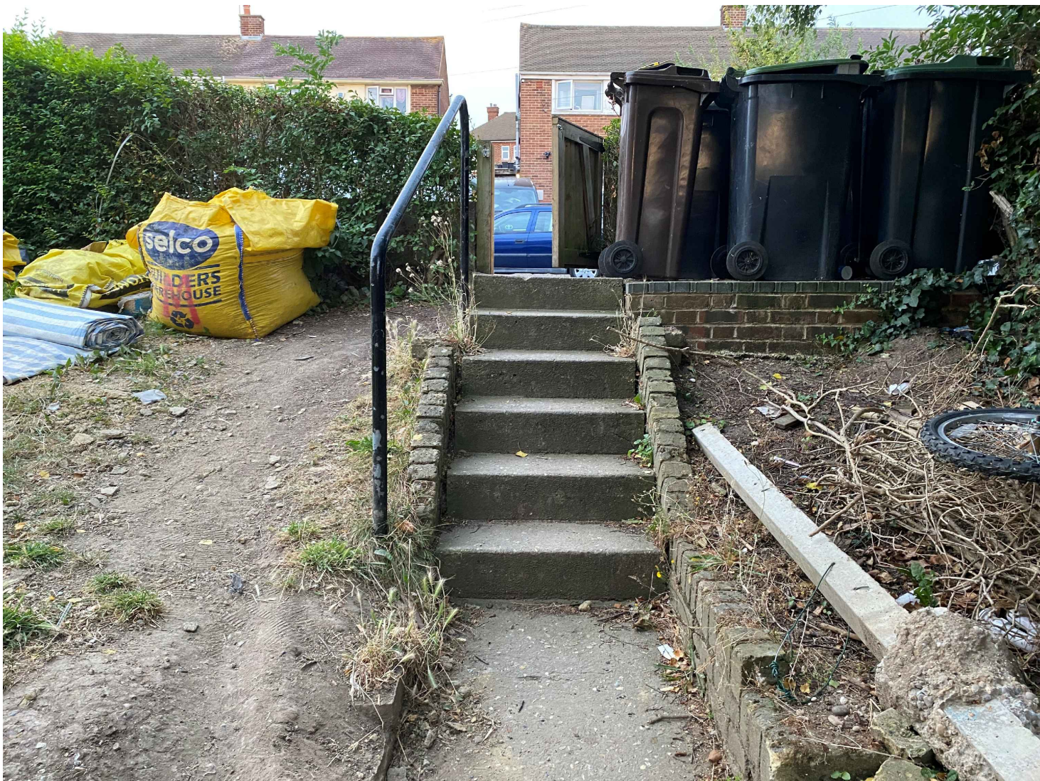
Photograph 04 View facing South-East, showing the level difference from street level down to the property. The bins can be seen on the right of the image where they are kept on a small plinth. This area is overcrowded which makes it difficult to reach the bins at the back, especially with the drop at the steps and the side of the plinth.
