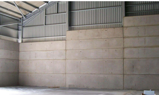
Example Image of Concrete Panels at the Base of the Barn
