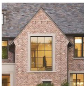
Stone Surround to Aluminium Windows
