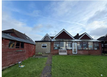
Fig.4 - Rear elevation of site showing existing extension
