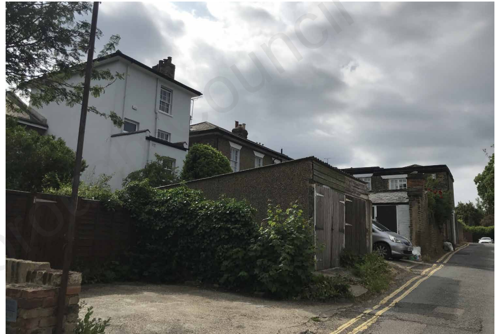
02. As demonstrated above, the properties are of varying materials, appearance, proportion, and arrangement. With this, there is no consistent design style apparent along the back of the properties.
