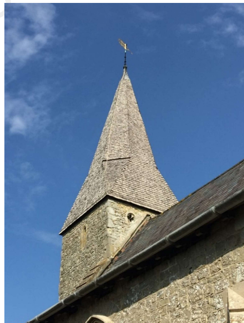
The same spire two years later (summer 2020), the oak having weathered to a typical silver-grey colour
