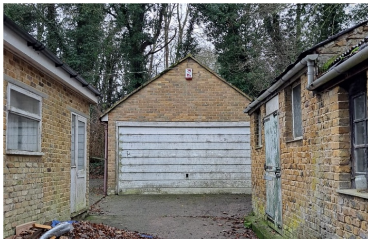
Building A (centre). Building B is on the right-hand side and Building C (not proposed for demolition) is on the left-hand side
