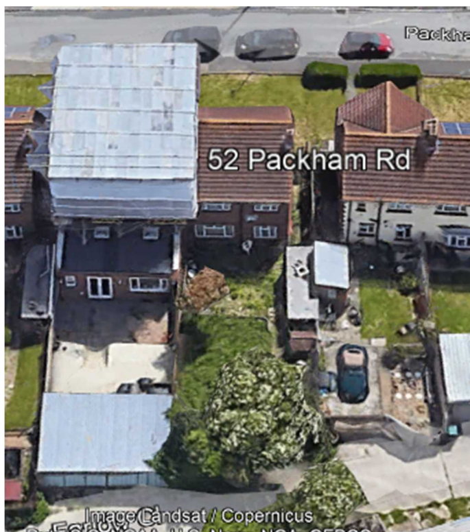
View of existing outbuilding:
