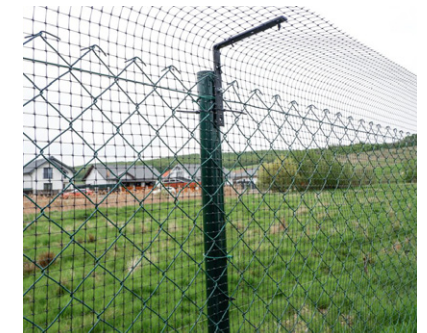
Provision of cat-proof fencing at the boundary adjacent to the SSSI
