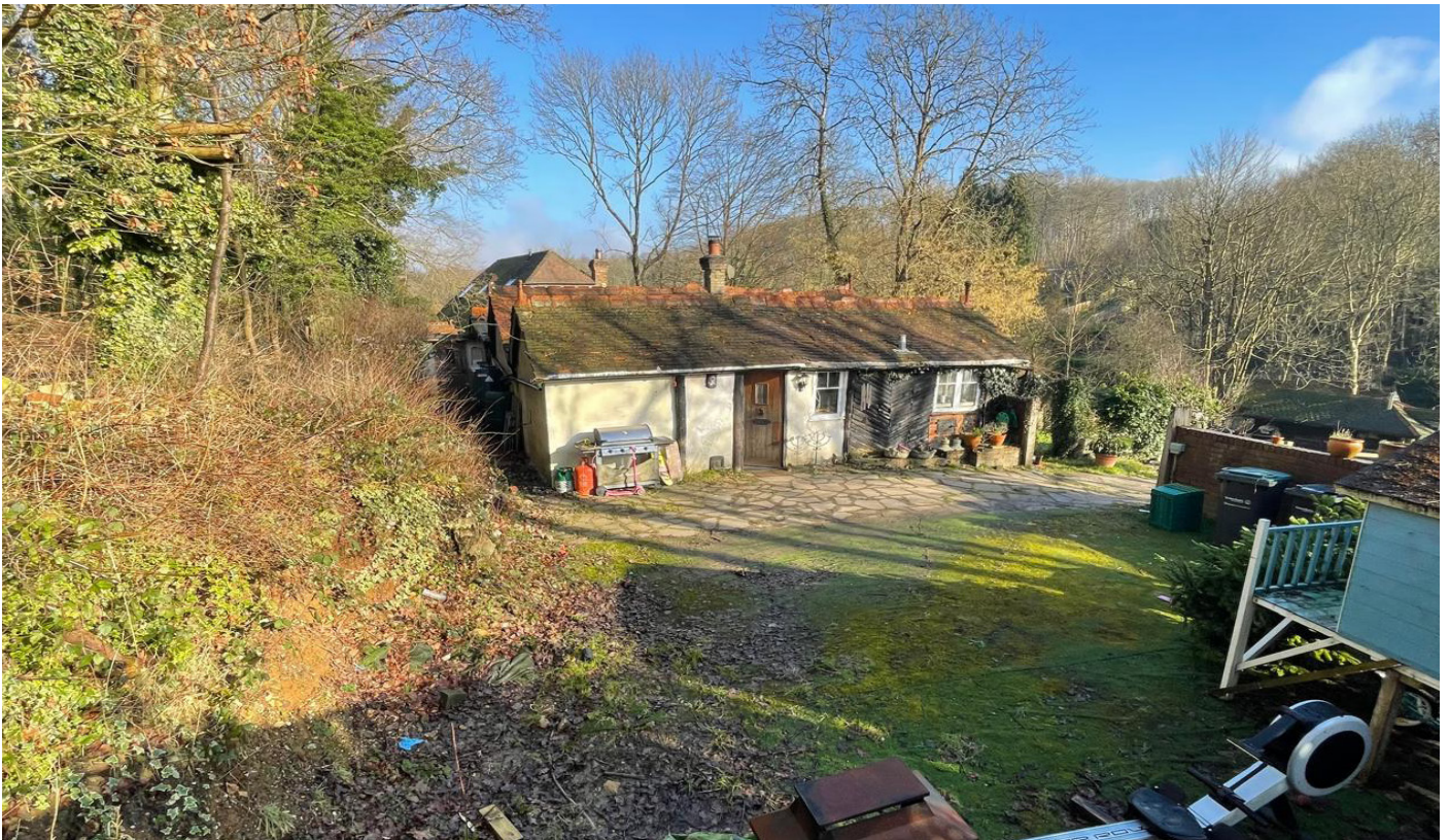
View North to Dwelling
