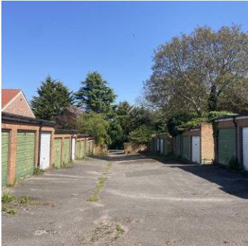
Figure 8: View of the site looking east.
