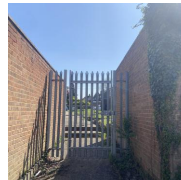
Figure 6: View of access to and from the site, looking south.
