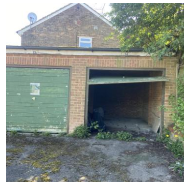
Figure 5: View of garages within the site.
