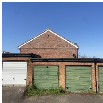
Figure 4: View of garages within the site.
