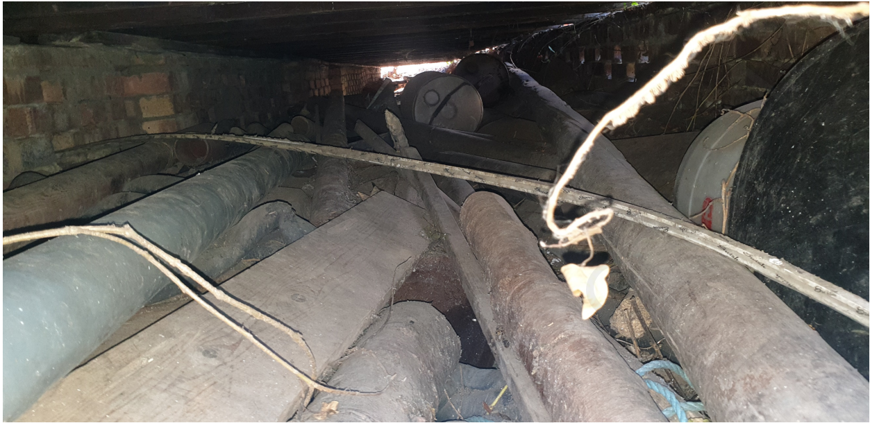
Figure 6: View of part of the partitioned void beneath the shed
