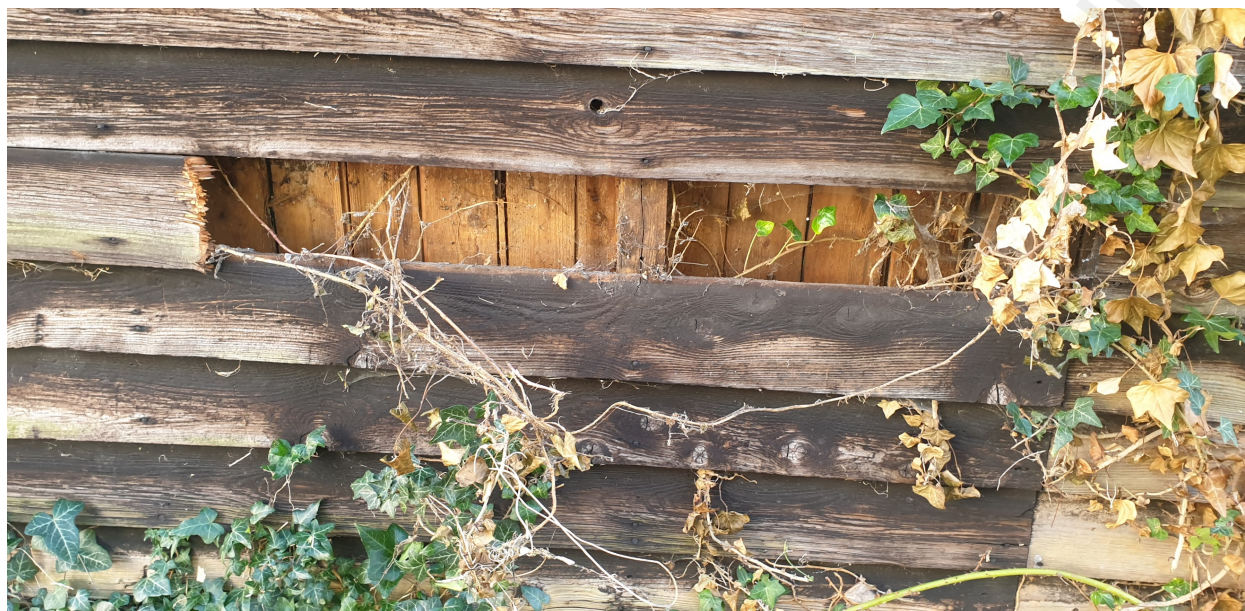
Figure 10: loose boards removed for inspection of the cavity between wall coverings
