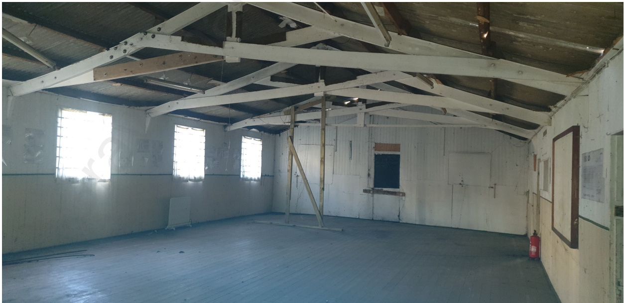
Figure 7: view of the main hall
