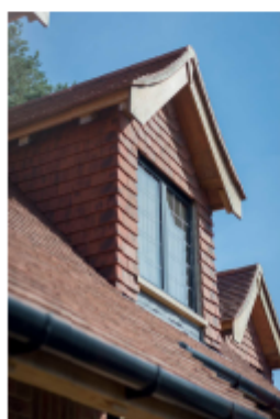
12 DORMER HANGING TILES IN RED TO MATCH THE RED CLAY ROOF TILES
