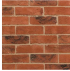
② WIENERBERGER OLDE HERITAGE BRICKWORK IN FLEMISH BOND
