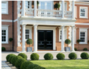
⑧ PRE CAST STONE WORK WITH PAINTED TIMBER SASH WINDOWS IN GLOSS GREY
