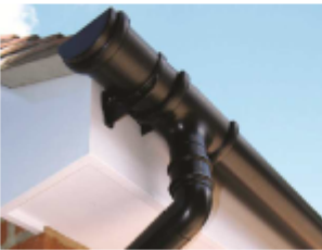
⑨ GUTTER - BLACK ROUND CAST IRON GUTTER AND WHITE SOFFIT AND FASCIA
