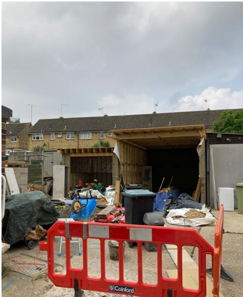
Front view of the new garage building
