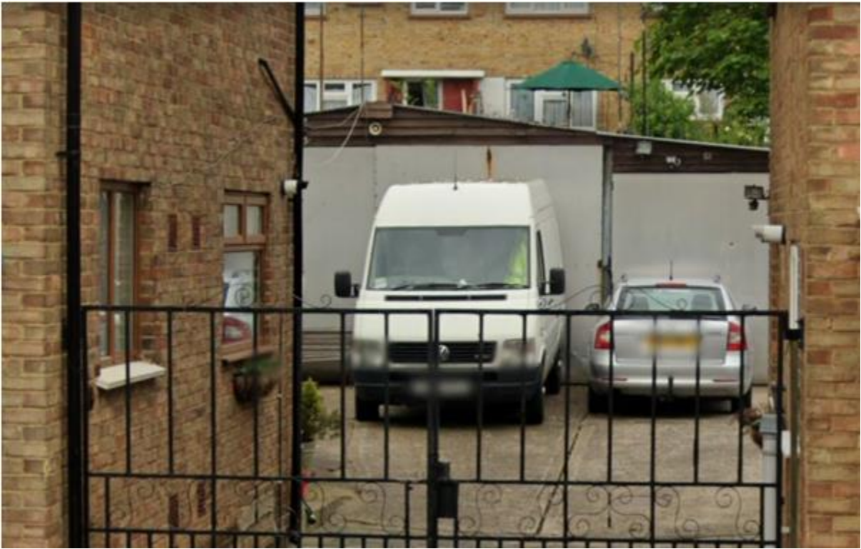
Front view of previous garage outbuilding
