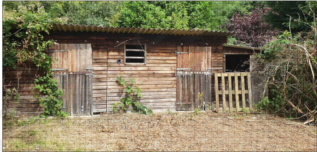
Existing Stable Block
