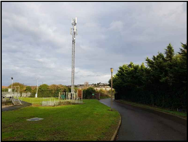
EXISTING SITE PHOTO
