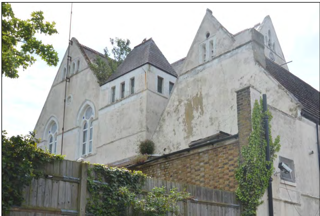
Plate 15: The north end of the east elevation showing the contrast in the rendered finish to the principal buildings and the exposed Flemish bond brickwork of the WC block
