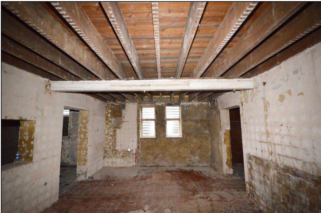
Plate 53: The western of the two rooms flanking the stair hall at the east end of the school looking north towards William Street
