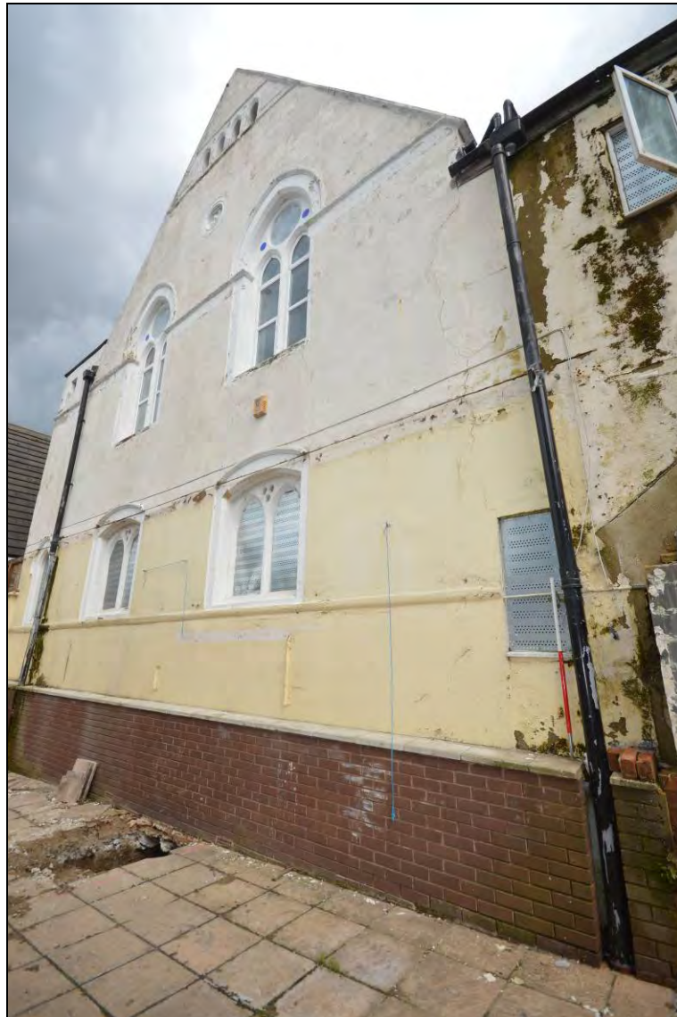
Plate 20: The west aisle
