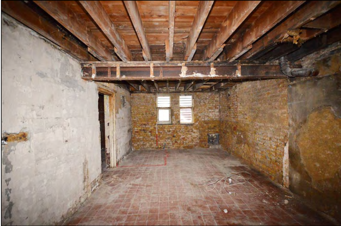
Plate 52: The eastern room on the lower ground floor, looking north towards William Street
