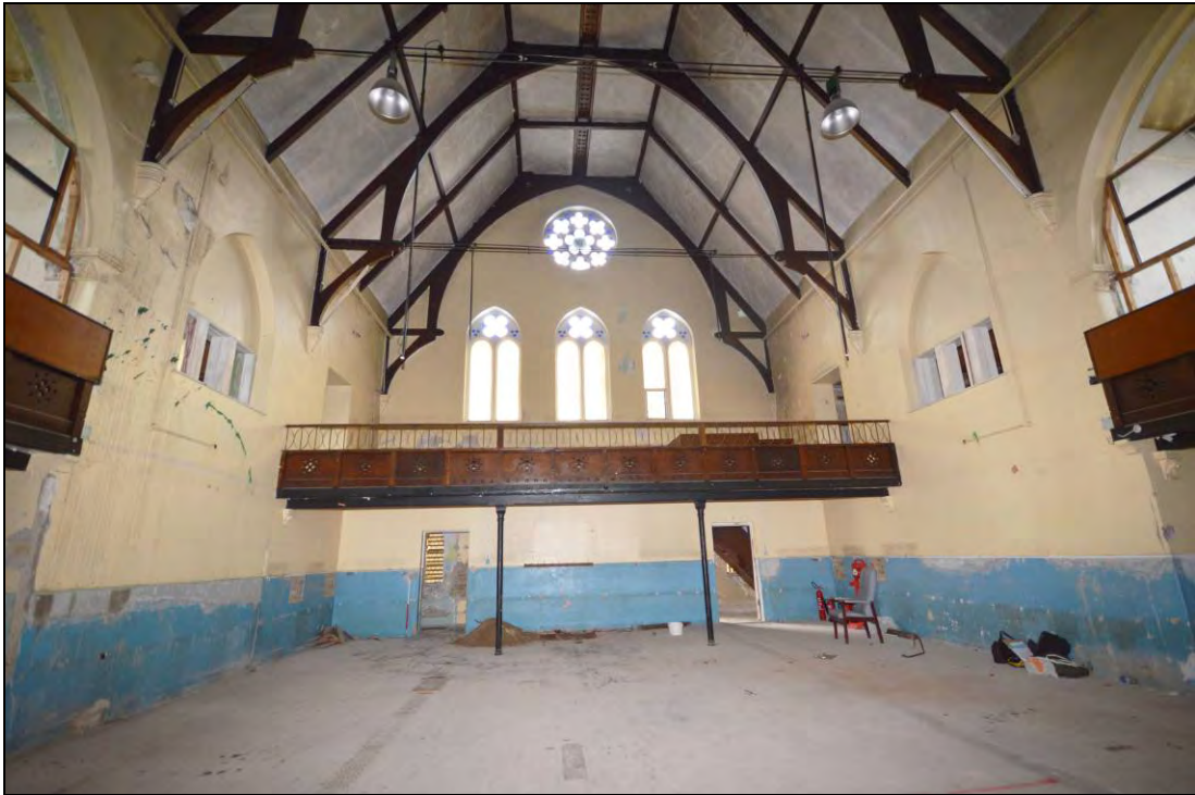
Plate 27: The nave looking south towards the gallery and entrance areas
