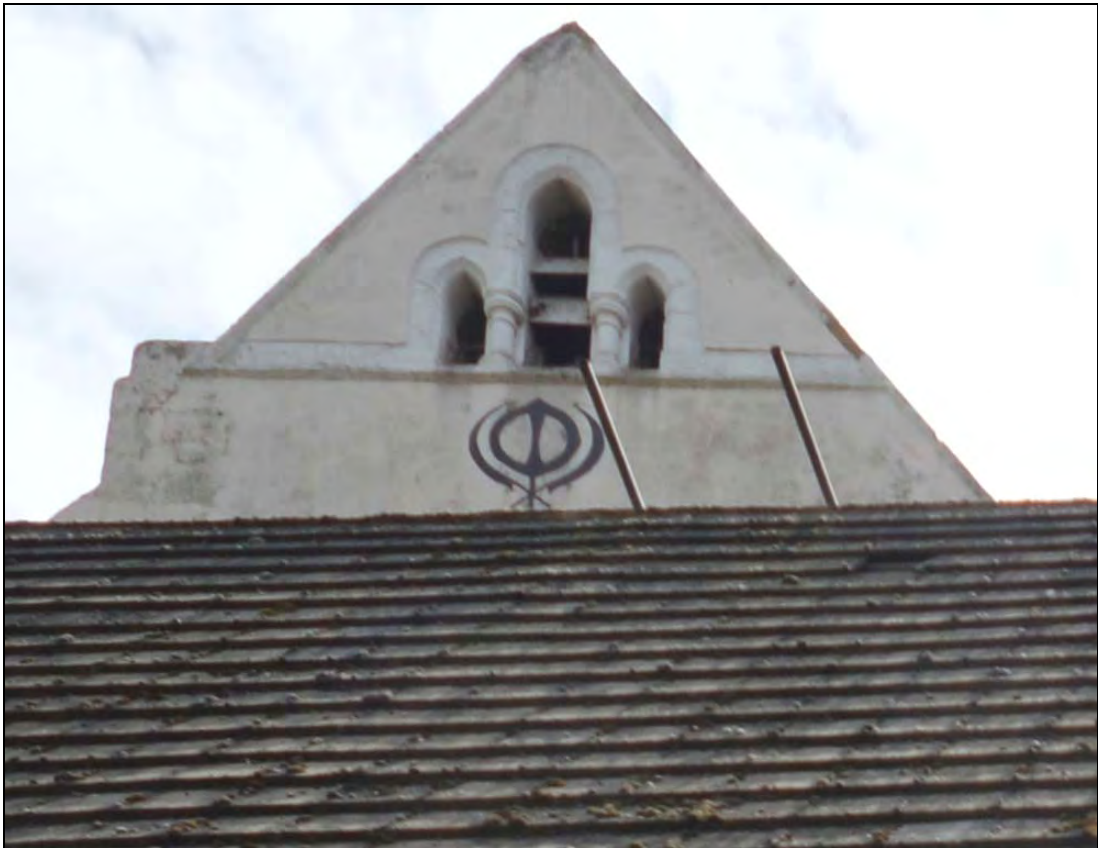
Plate 13: The north gable of the church
