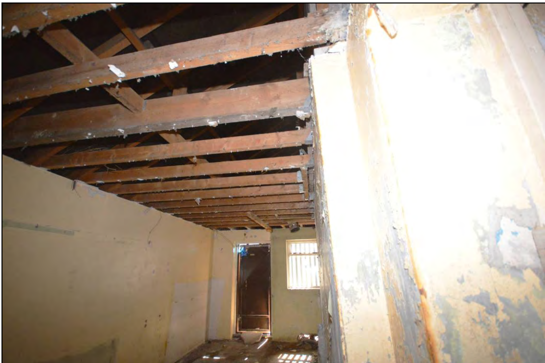
Plate 57: The interior of the porch extension added to the east side of the church in 1982, looking south
