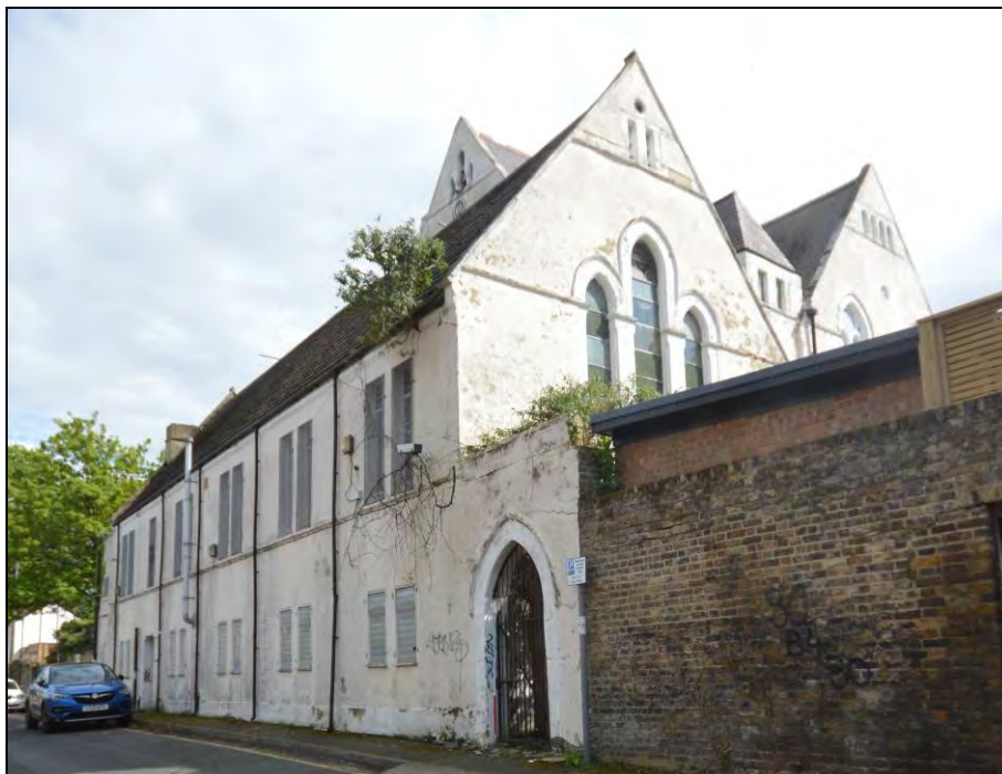
Plate 18: The west end elevation of the school, stair turret and west aisle from William Street
