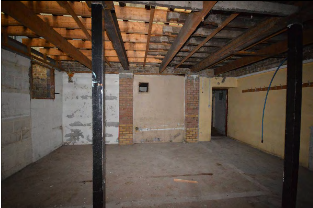
Plate 54: The room below the northeast corner of the nave looking north towards the doorway leading to the stair hall at the east end of the school
