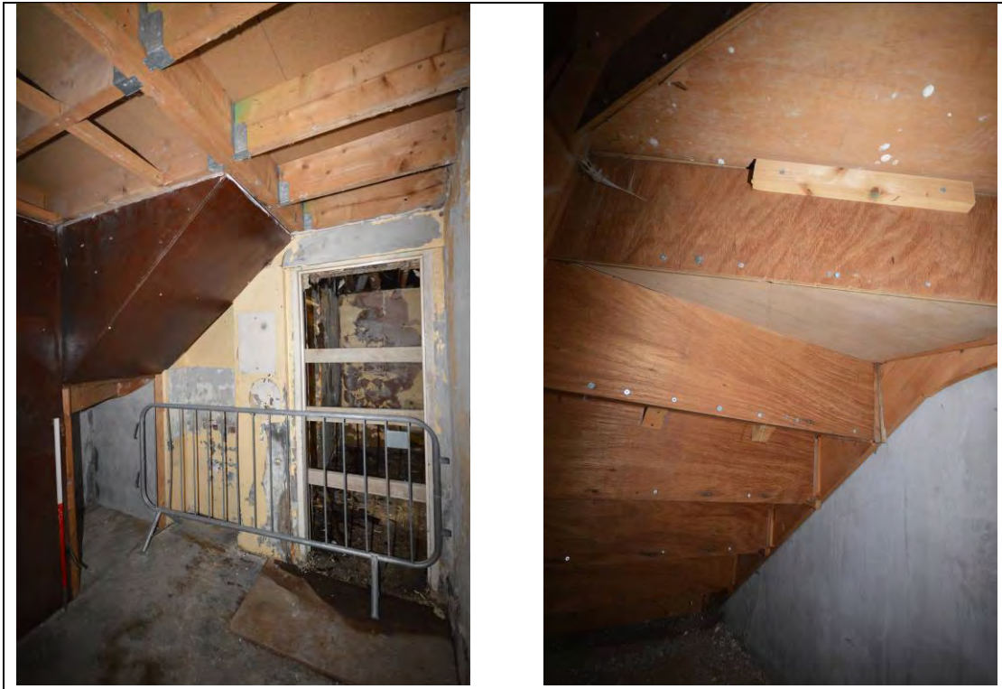
Plate 43: Detail of the inserted floor and the staircase structure and a doorway that had led into the neighbouring single storey utility lean-to
