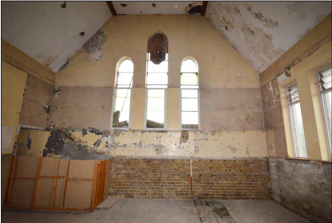
Plate 39: The tripartite feature window at the west end of the school room on the upper ground floor, contrasting with the plain window openings in the north elevation
