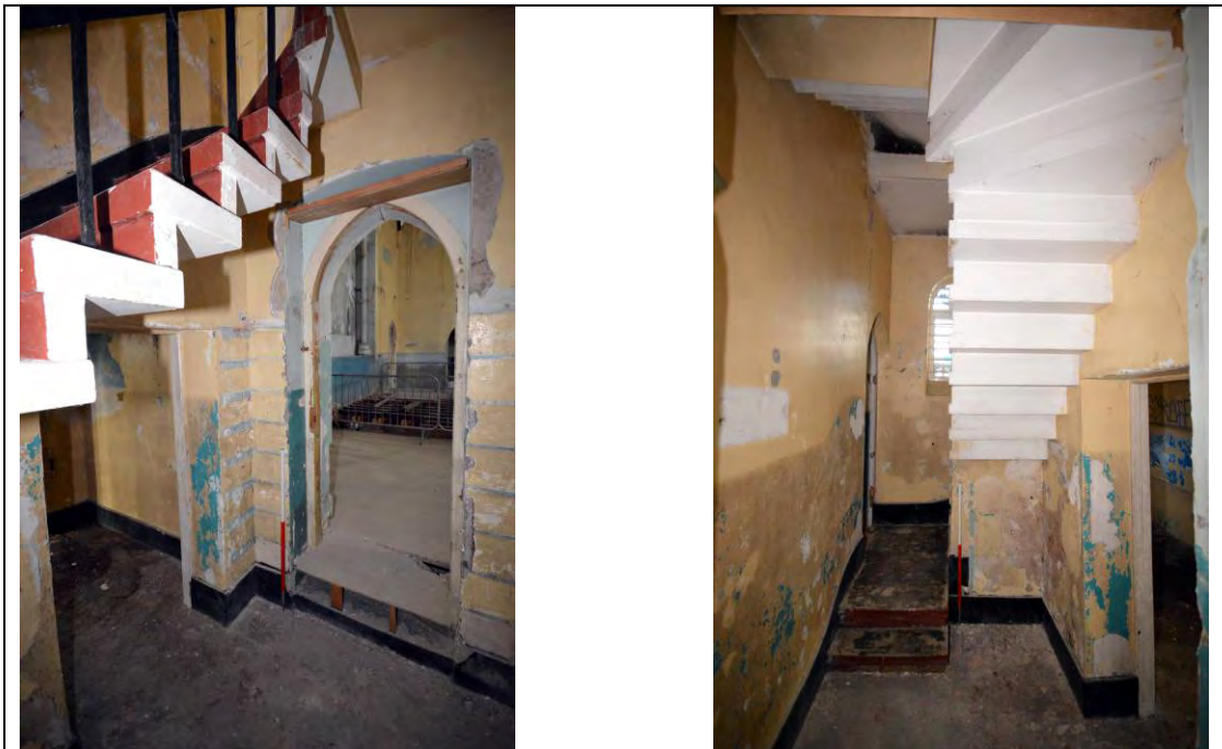
Plate 37: Details of the stair turret staircases
