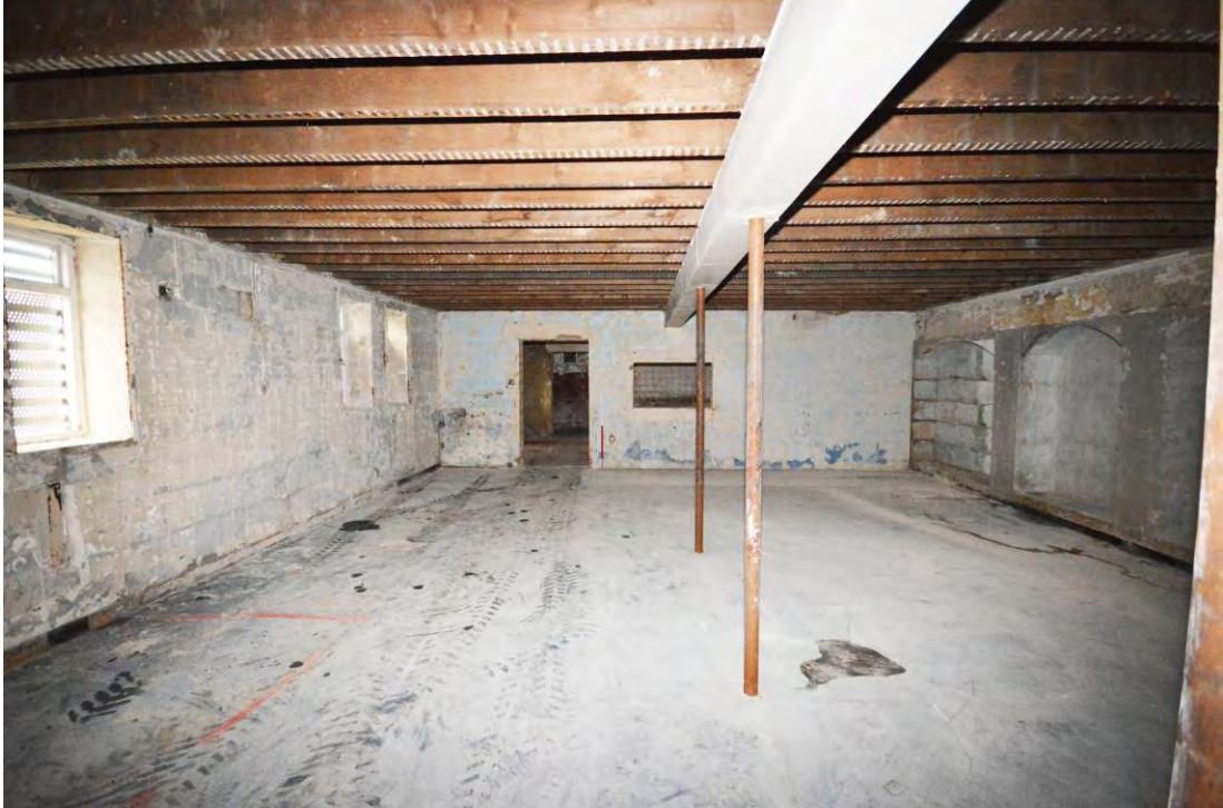
Plate 48: The lower ground floor classroom at the west end of the range looking east
