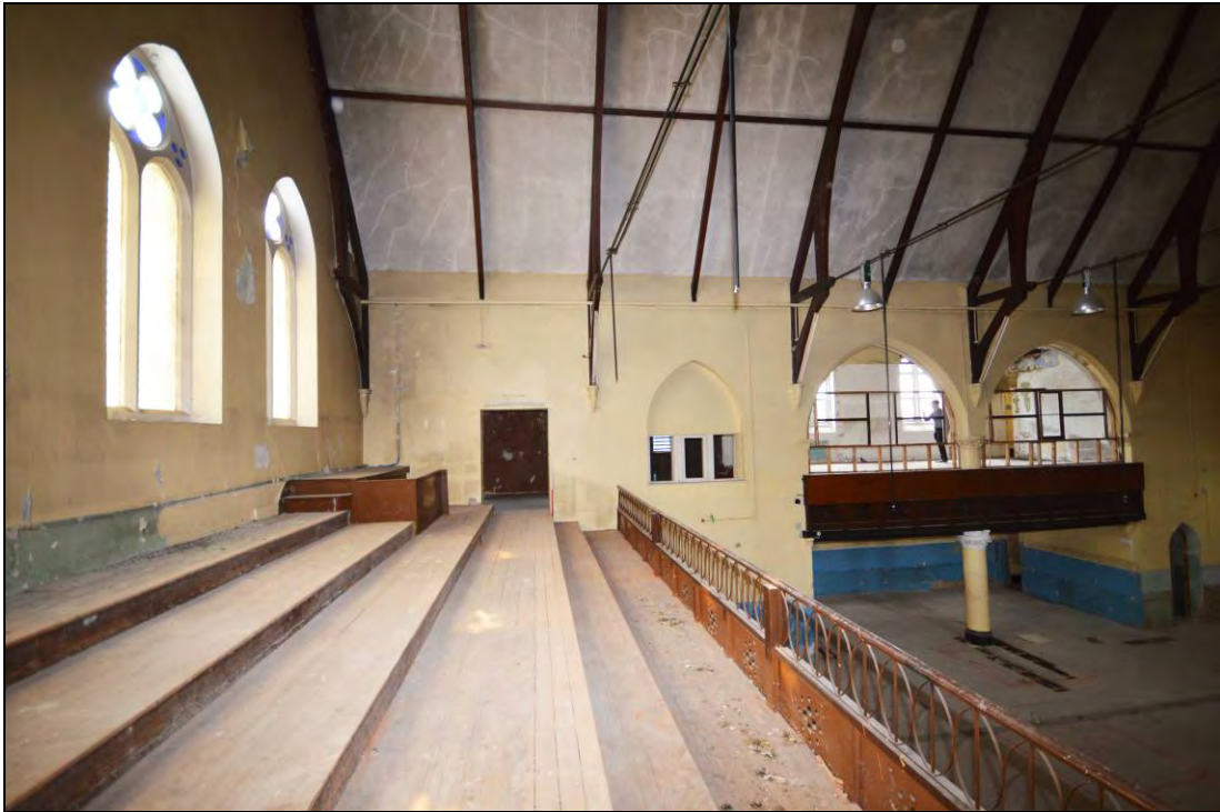
Plate 34: The west side of the south gallery showing the staircase and the entrance inserted into the west wall to link the aisle to the first floor extension added in 1975
