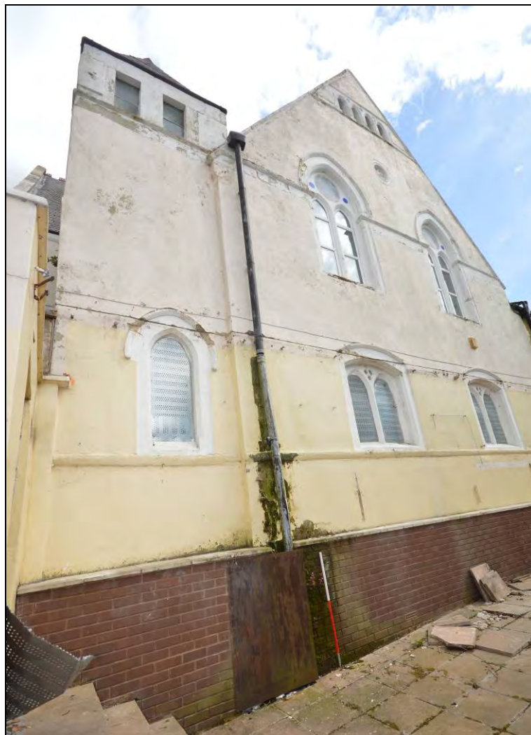
Plate 19: The west side of the building showing the stair turret and west aisle
