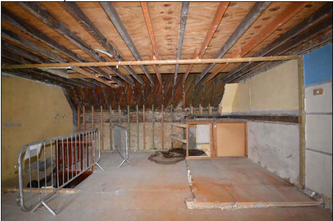
Plate 46: The south side of the eastern rooms at the modern first floor level looking towards the sharking boards laid over the rafters
