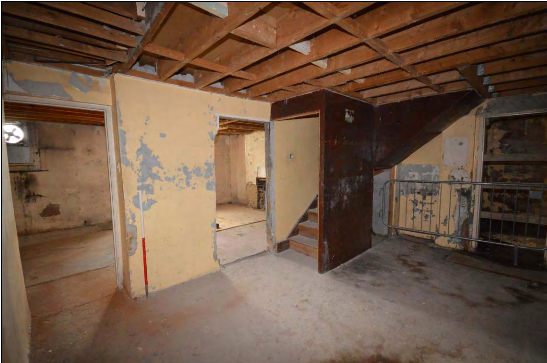
Plate 42: The interior of the eastern group at the end of the school house: the doorway to the west is in the location of the original; the partition adjacent, doorway, staircase and ceiling structure are the result of 20 th century alterations
