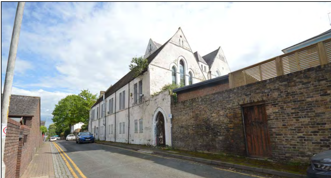
Plate 64: The William Street side of the property looking east
