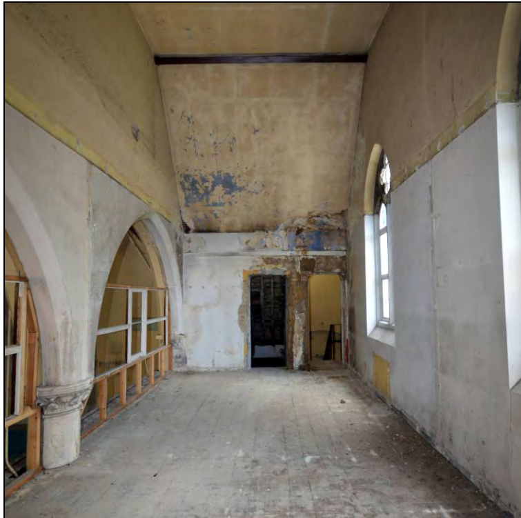
Plate 32: The north end of the east gallery showing the interior, the later in-fill of the arcade and the access to the stair turret
