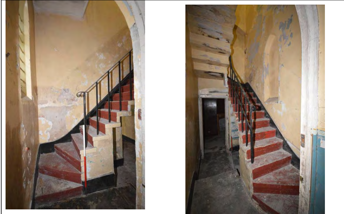
Plate 36: The west and east staircases accommodated within their own purpose-built stair turrets
