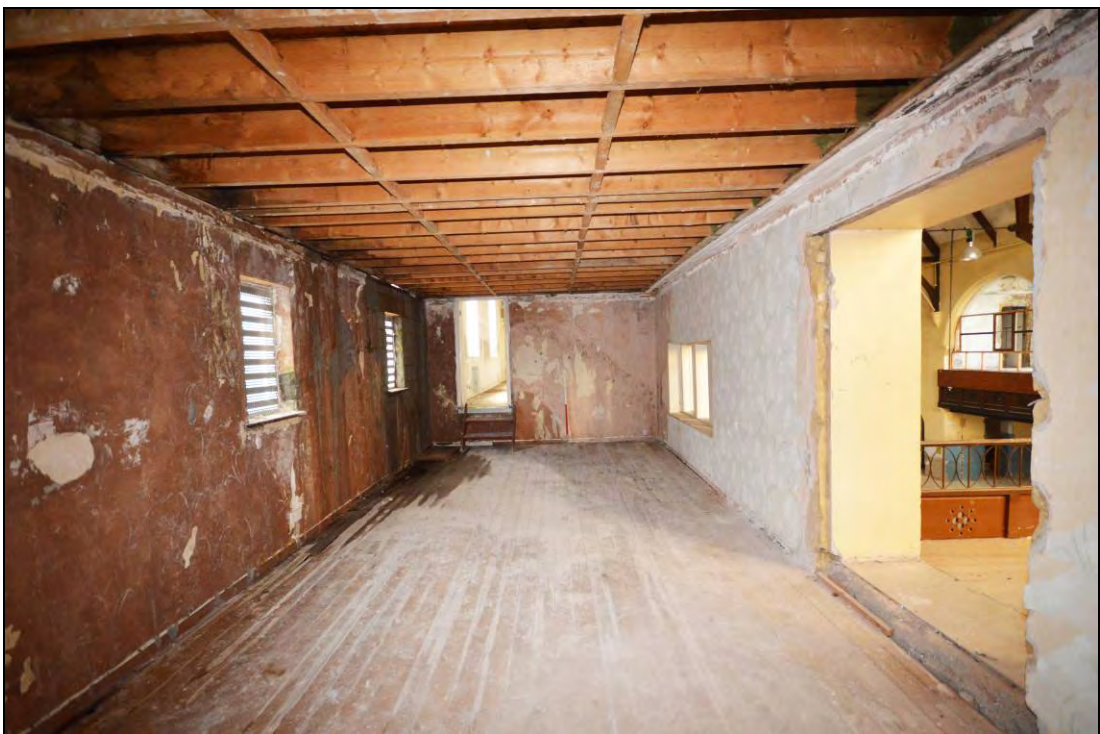
Plate 60: The interior of the southwest extension looking north towards the doorway created in the south wall of the west aisle to link the two parts
