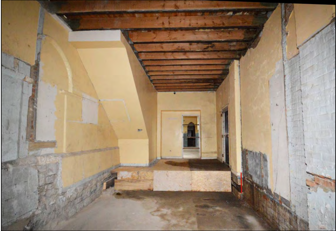
Plate 59: The interior of the southeast extension looking north towards the staircase accessed from within the aisle. Note the blocked pointed-arch-headed window in the west wall
