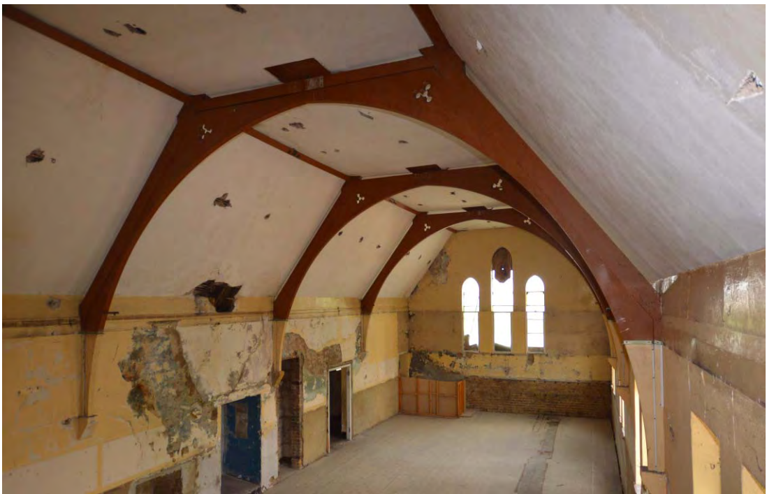
Plate 41: The roof structure over the school classroom on the upper ground floor looking towards the west end of the range
