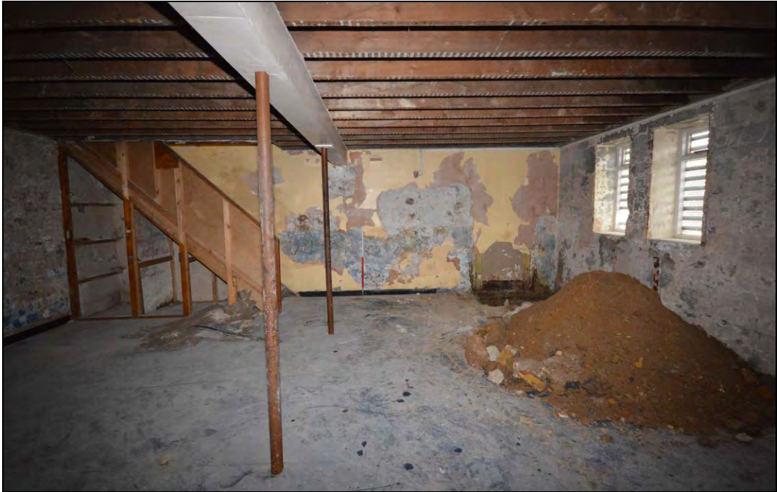
Plate 50: The west end of the main classroom on the lower ground floor looking west towards the inserted staircase and blocked doorway
