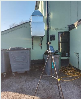
ST1 monitoring position
