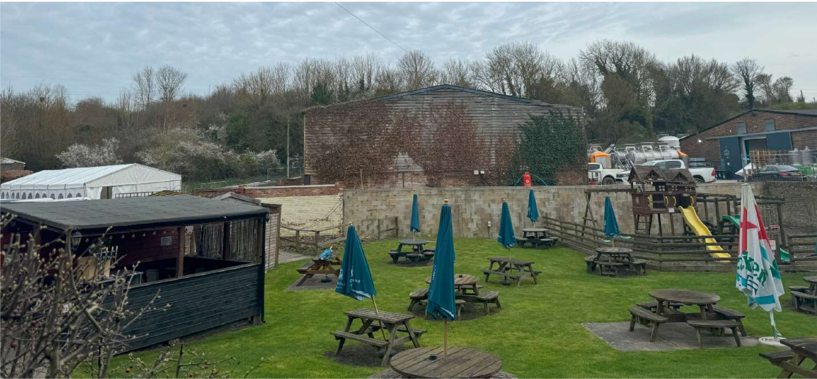
1_ The rear garden of the pub showing the agricultural buildings in the context of the pub and the poor quality boundary wall.
