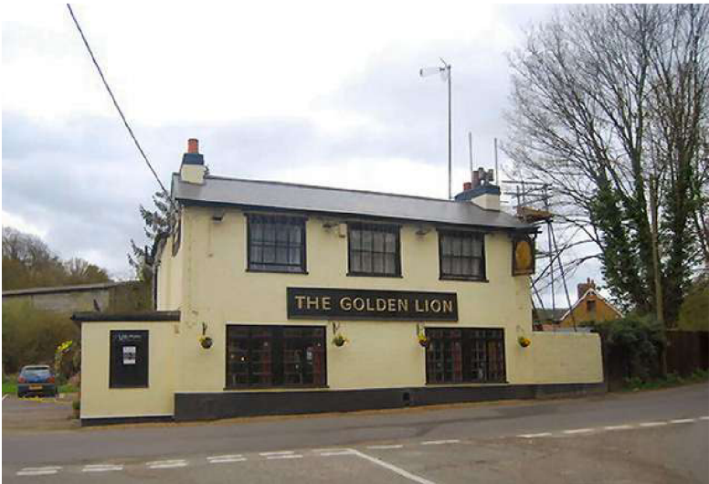
Recent photo showing terrace removed, new W.C. extension and infilled front door
