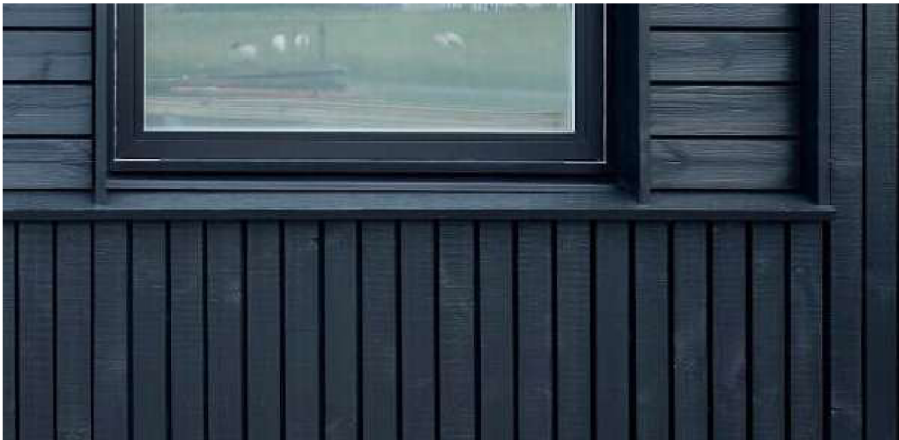
Example of black timber cladding proposed for the new extension
