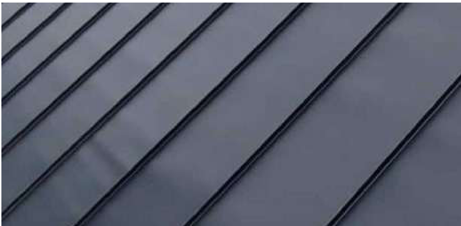
Zinc standing seam roof
