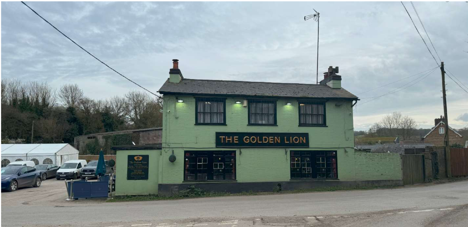
1_ The front elevation of the building with former entrance door infilled. Low quality boundary treatments either side of the pub.
