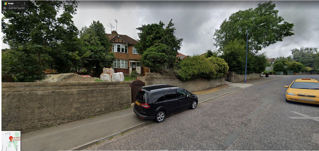
Picture showing 46 Whitehill Ln, Gravesend DA12 5LZ house and front retaining wall, which will be converted into parking space. Property has descent size front land, which can use for parking purpose. Front retaining wall to be reconstructing using similar materials to match existing. No garage doors to be installed.
