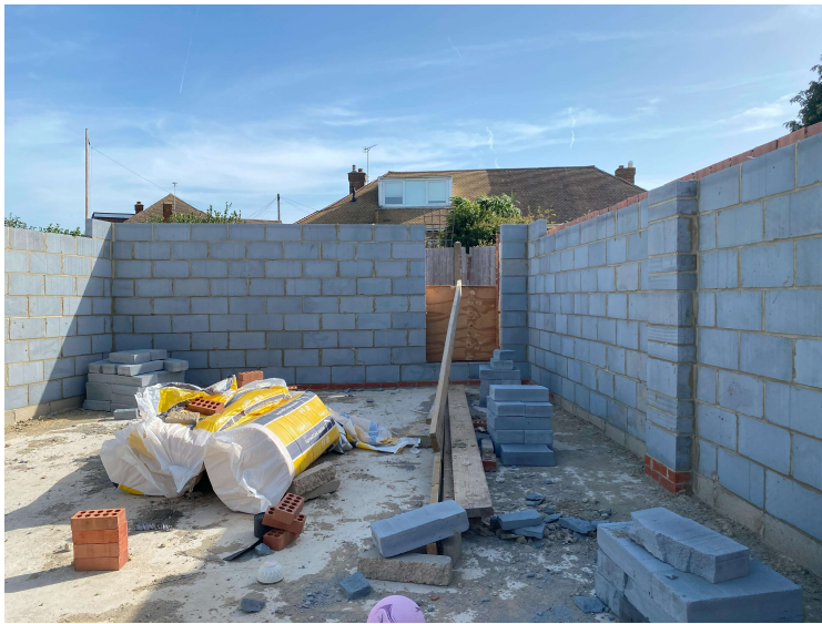
Existing construction stage of the rear games room
