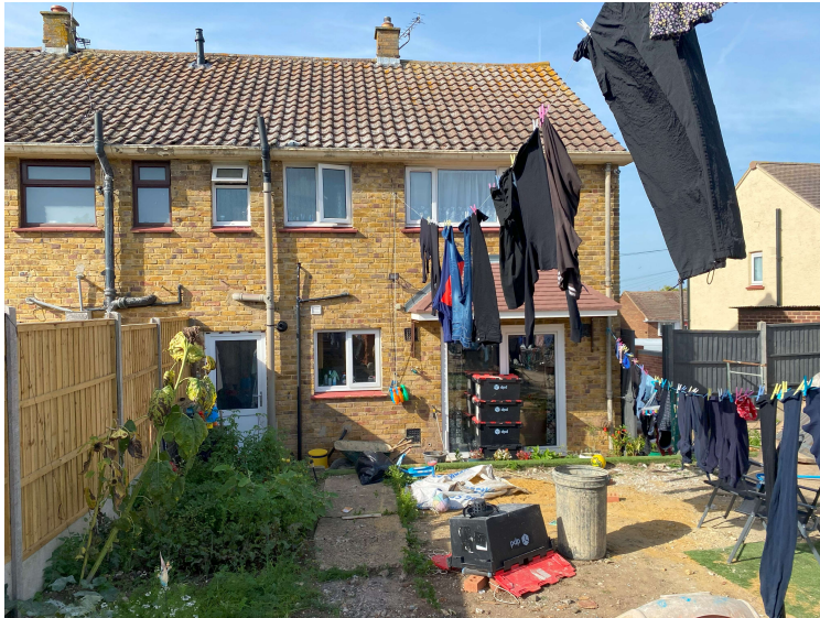
Existing rear elevation of the main dwelling
