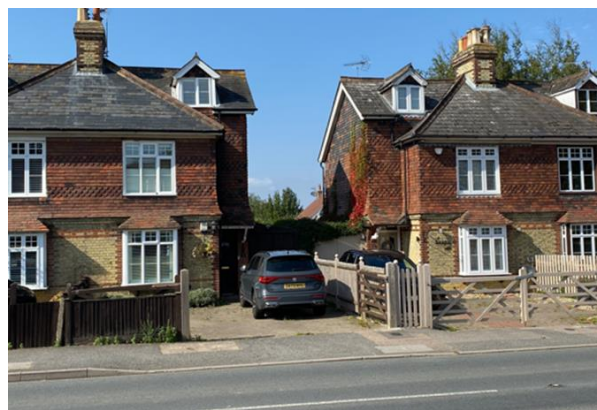
View between 2 and 3 Sunnyside, Wrotham Road
