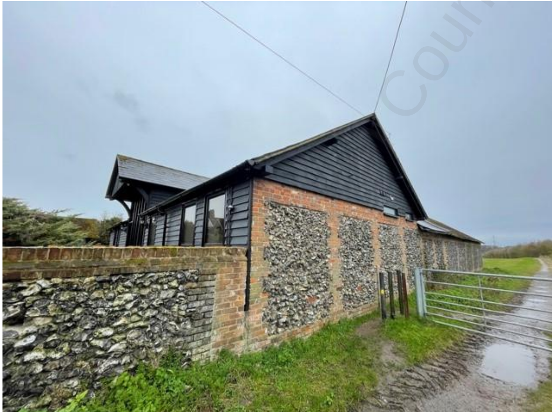
Fig 2.1: View of north elevation flank wall adjacent to public footpath with attached barn to the rear.
