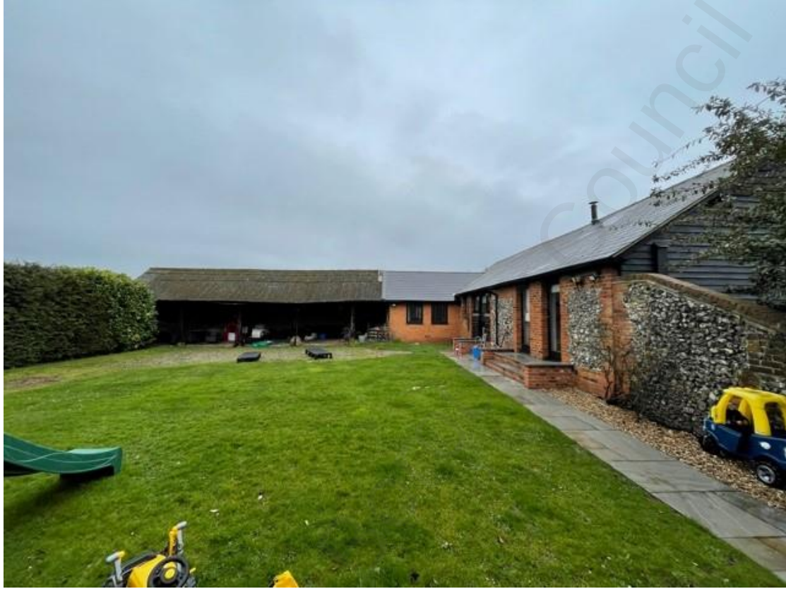
Fig 1.2: The barn (left of image) is attached to the main dwelling, forming an L-shaped building'. The barn is timber frame, open to the garden with a corrugated roof (assumed to be asbestos) and a flank wall to the side boundary of red brick with flint infill. The barn is currently in a poor state of repair.
