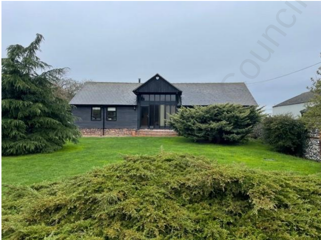
Fig 1.1: Front Elevation of the main dwelling 'The Barn' in Thong Lane, comprising black painted timber cladding, red brick plinth and asbestos tiled roof.
