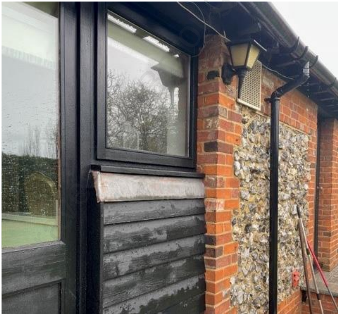
Fig 2.2: Existing main dwelling: red brick, black painted timber cladding and flint infill
