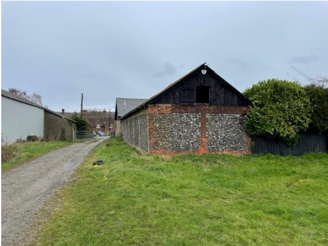
Fig 2.2: View of the rear elevation (W) of the barn, with public footpath to the left.
