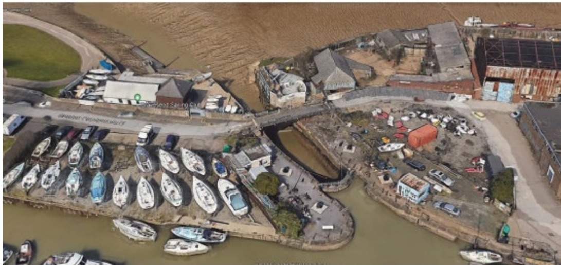
Figure 1. Aerial View of the Swing Bridge, Gravesend.
