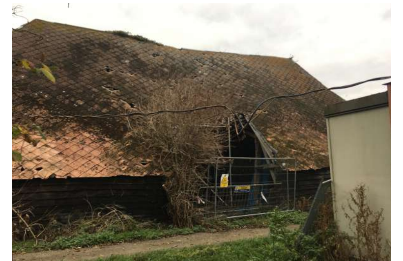
Kent barn south east elevation in winter
