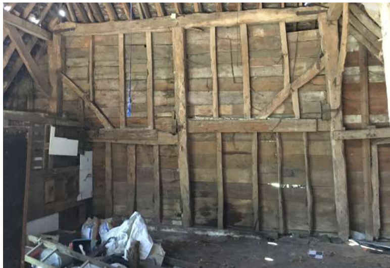
Kent barn - Internal framing
