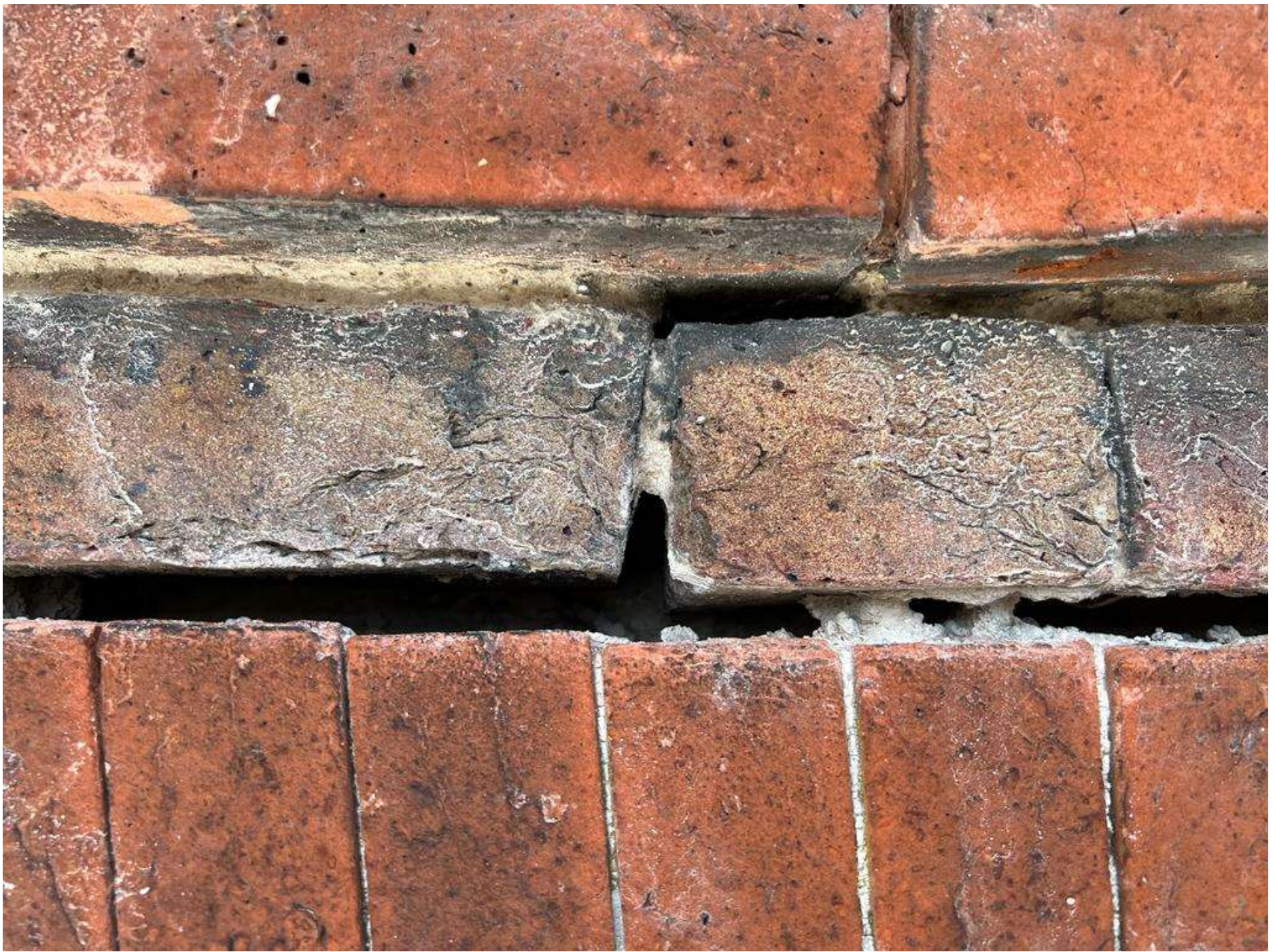
3. South elevation - above window detail
