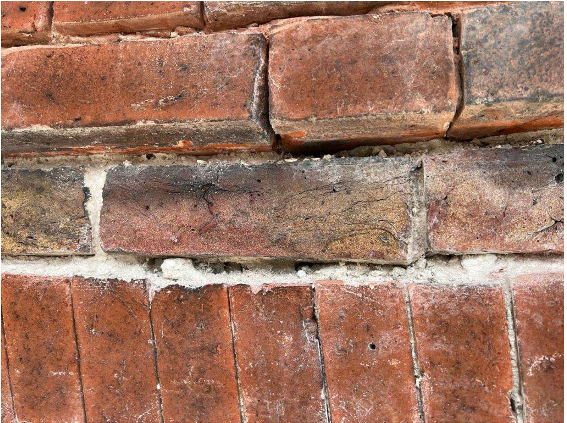
2. South elevation above window detail
