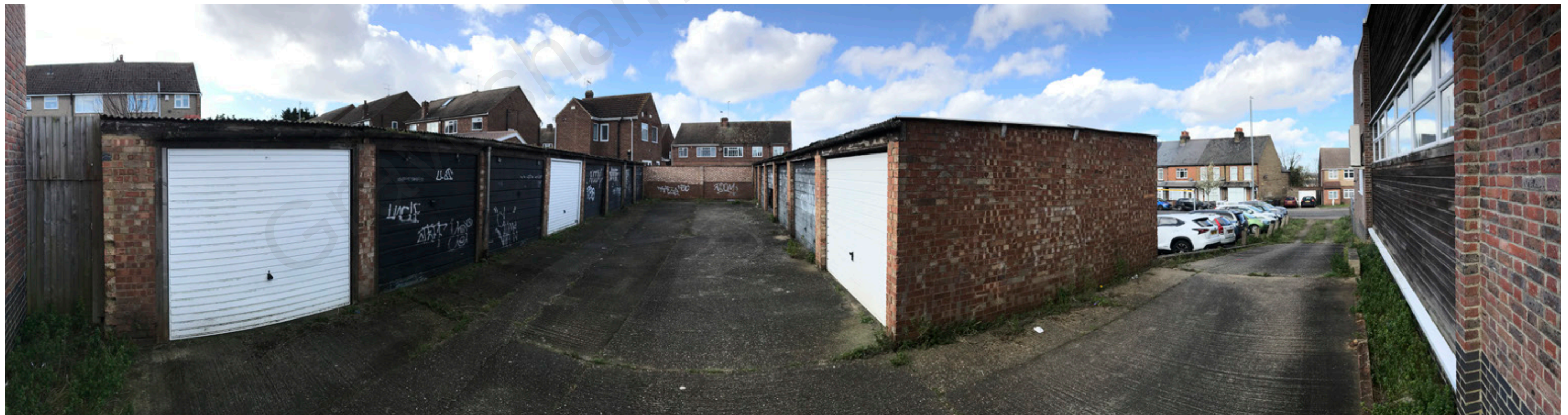
Panorama from entrance, across front of the existing garages, and looking out to the road
