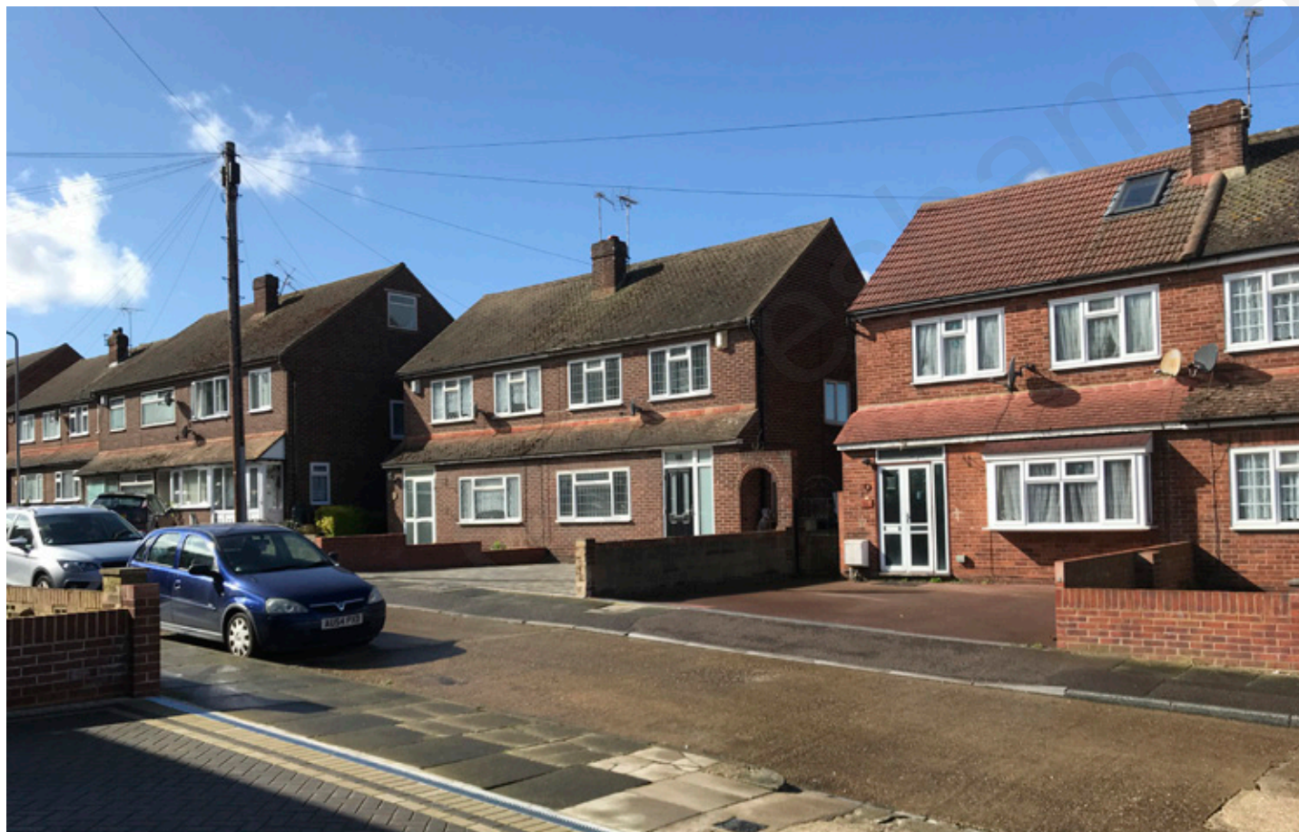
Osney Way - Two storey housing with pitched roof with room in roof
