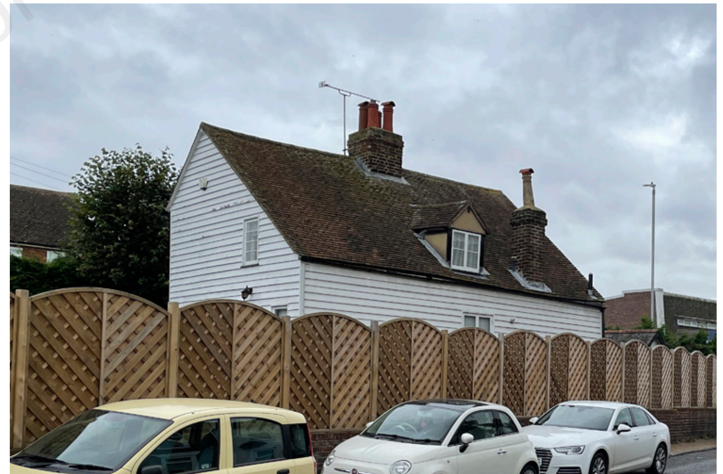
1 Chalk Road, featuring an asymmetric pitched roof with dormer and chimney
