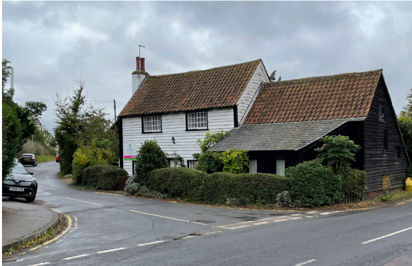
The Forge (Grade II Listed Building) 2021
