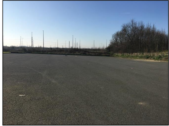
Photo 2: Hardstanding that covers majority of Site.
