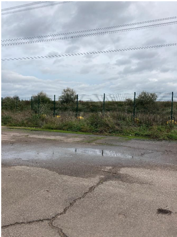
Photograph 3 – Hardstanding at Tilbury Site
