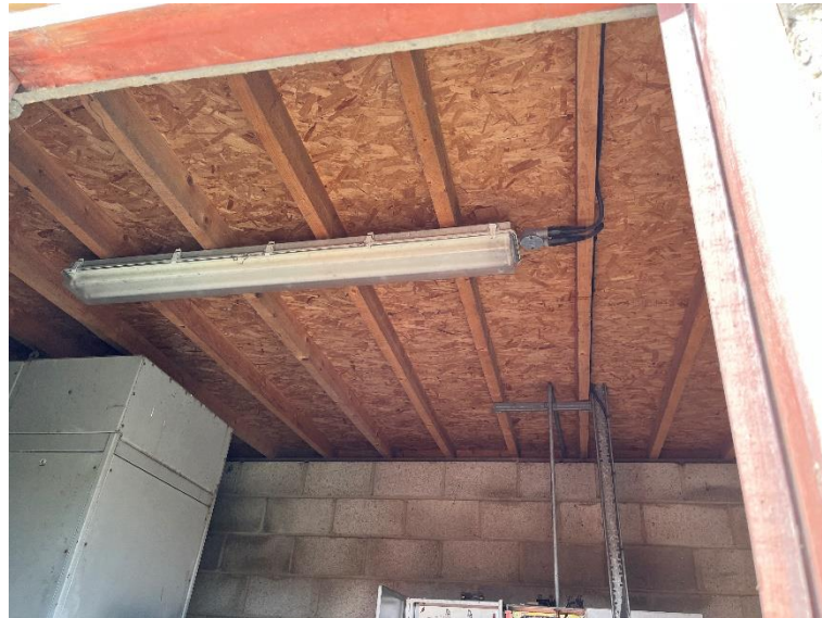
Plate 3: Interior of Building 1 open to the roof
