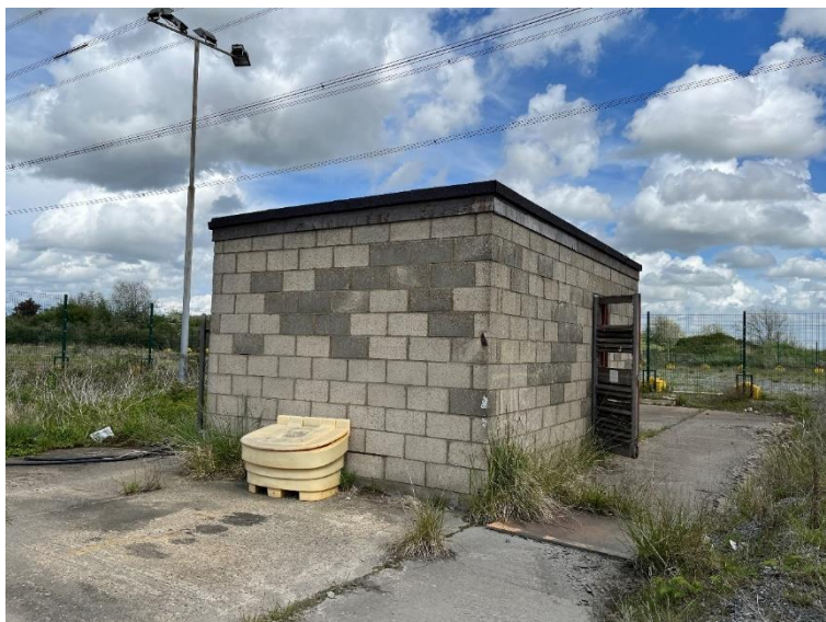
Plate 1: Building 1, looking north-east
