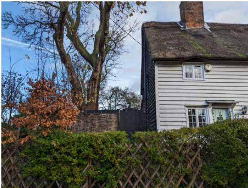
View from Church Street
