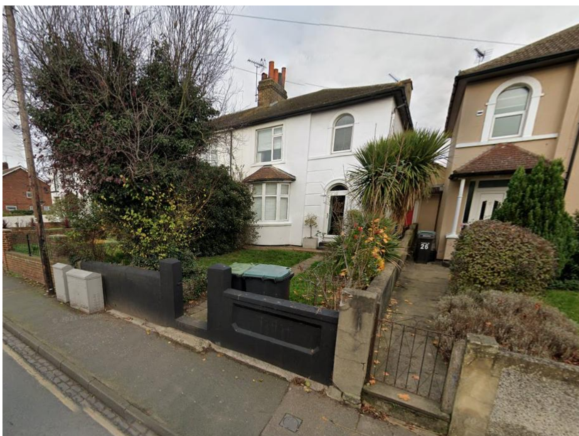
Image 2: Photograph of front elevation of property as viewed at street level
