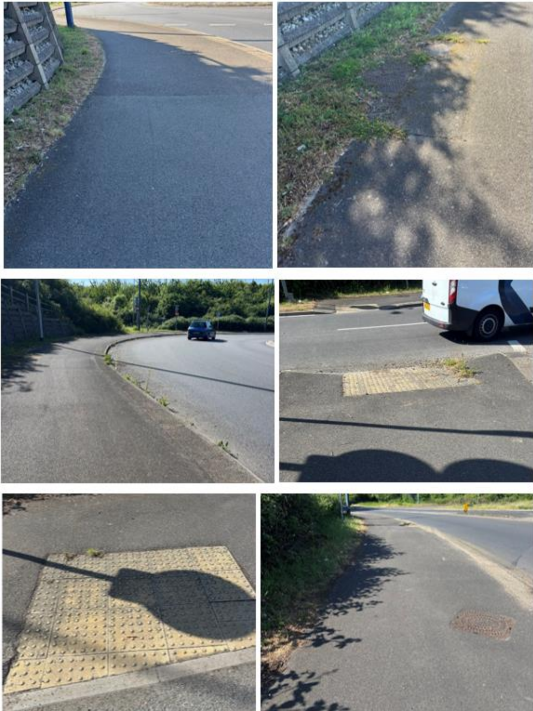
Figure 3.1 Existing Infrastructure – WCHAR Study Area
