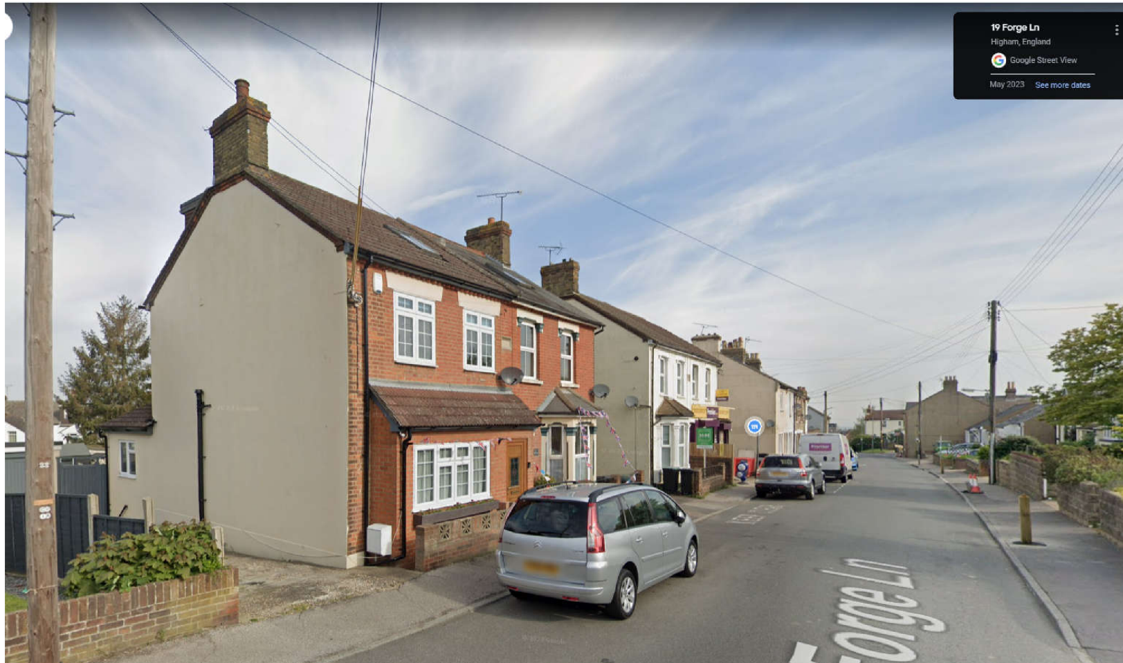
Photo 1 - No 24 Forge Lane Higham – Street View 2023
