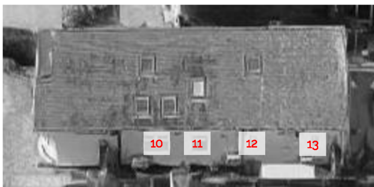
17 Malvina Avenue (Side Elevation)
