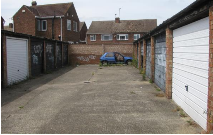
Inside the existing garage court
