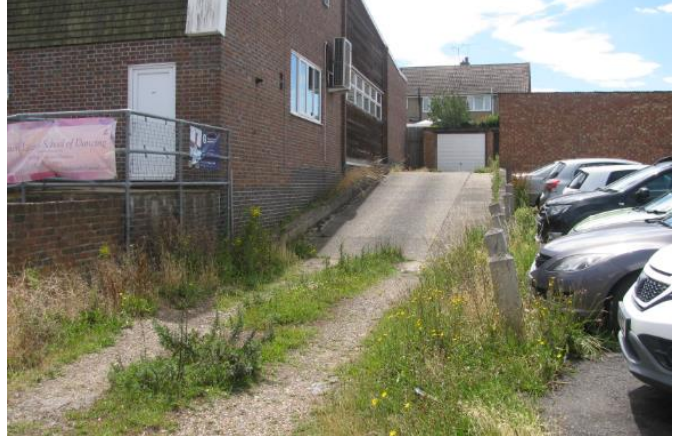
Ramped access to the garage court
