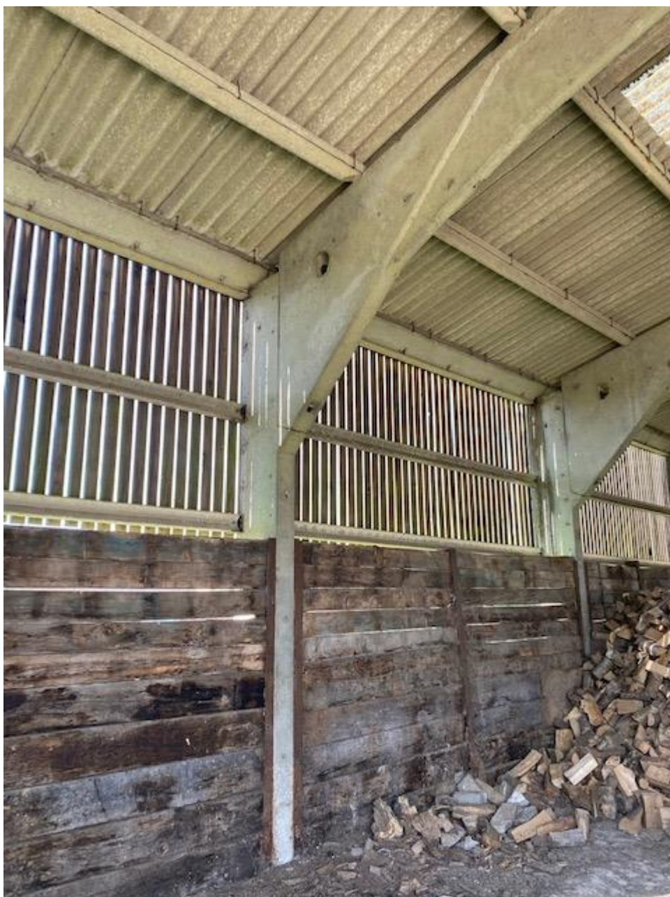
Existing Barn Viewed Internally
