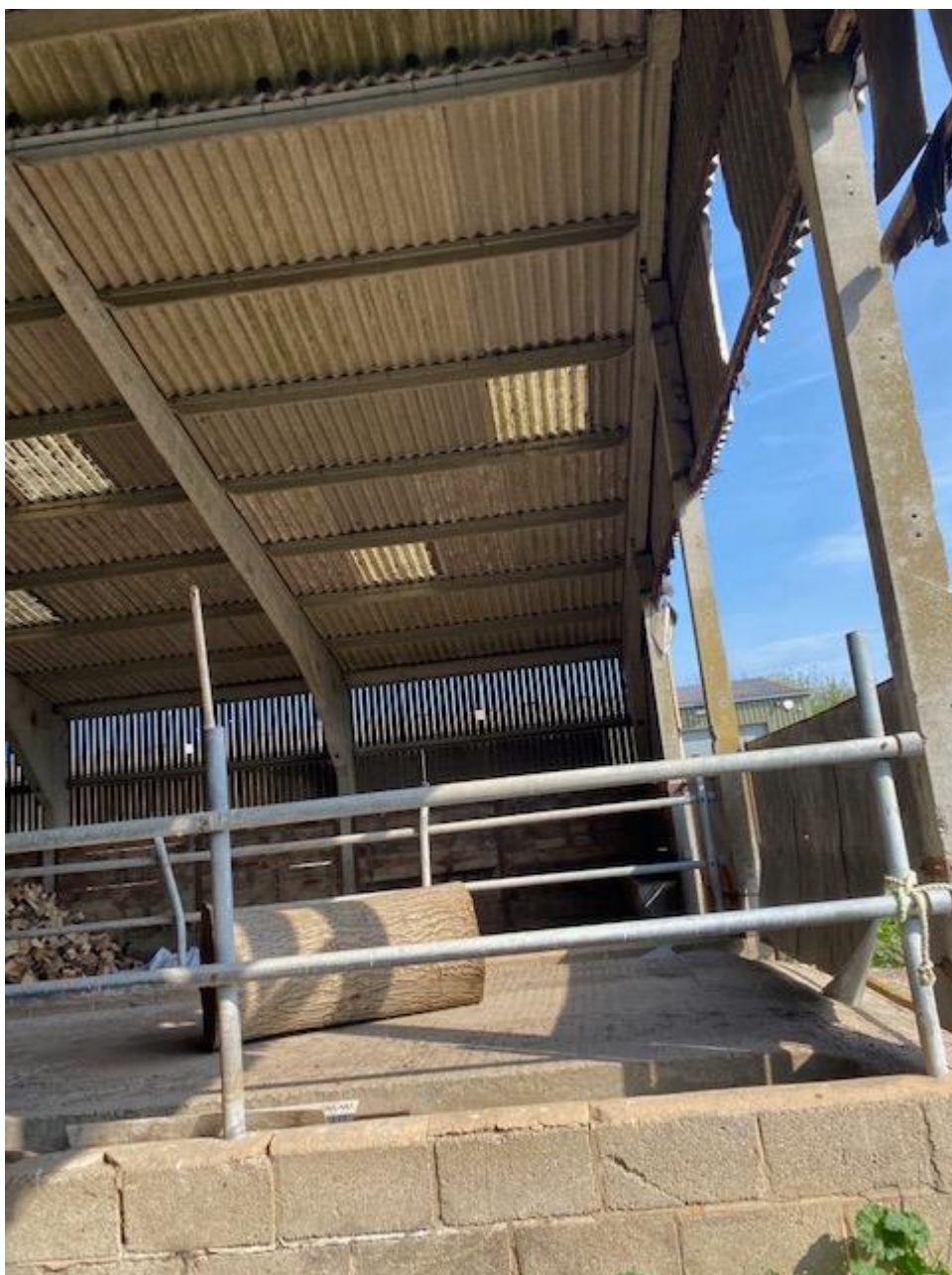
Existing Barn Viewed Internally
