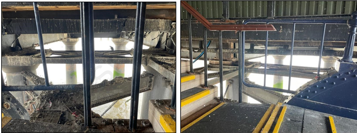
Figure 3: Existing condition underside of pier 1
