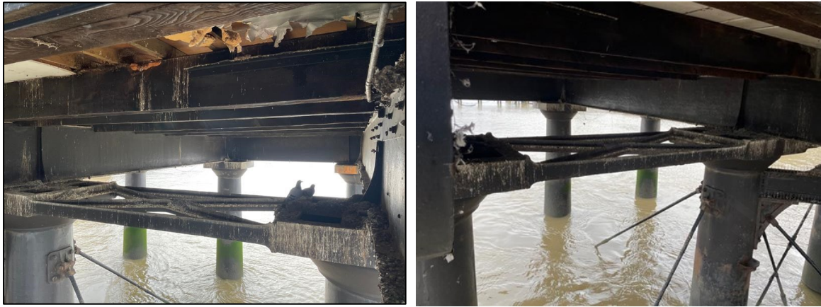
Figure 4: Existing condition underside of pier 2
