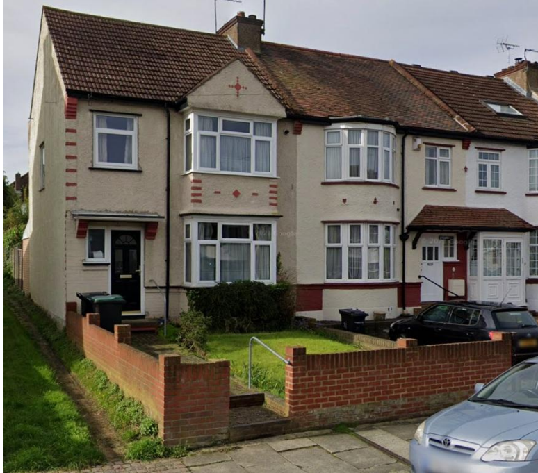
FRONT ELEVATION PRIOR TO COMMENCEMENT OF WORK
