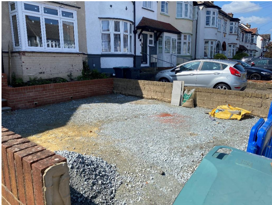
FRONT ELEVATION PRIOR AFTER COMMENCEMENT OF WORK
