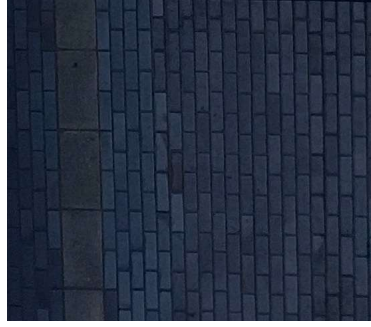
Existing brick work to gym
