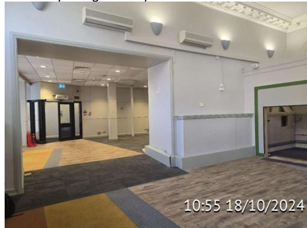
Photo 2: Ground Floor Structural Opening where partition wall will be installed:
