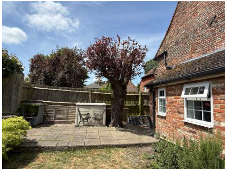
Fig 33-View of the modern boundary fence and hard paving.
