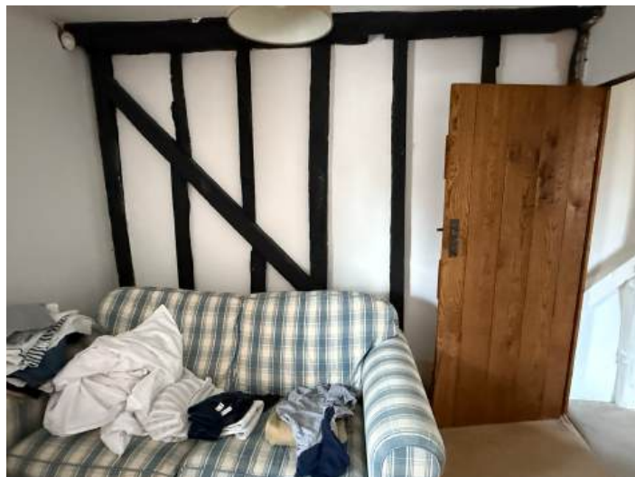
Fig 22–Stud wall from the 1940's in guest bedroom with 19thC door.
