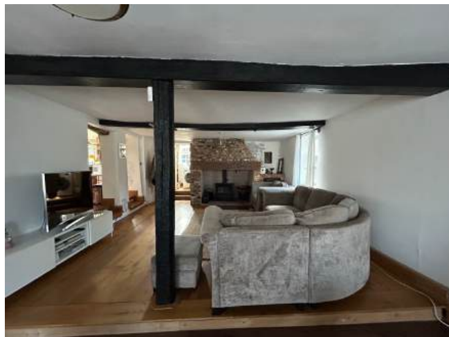
Fig 09 – Modern steel beam and timber post
