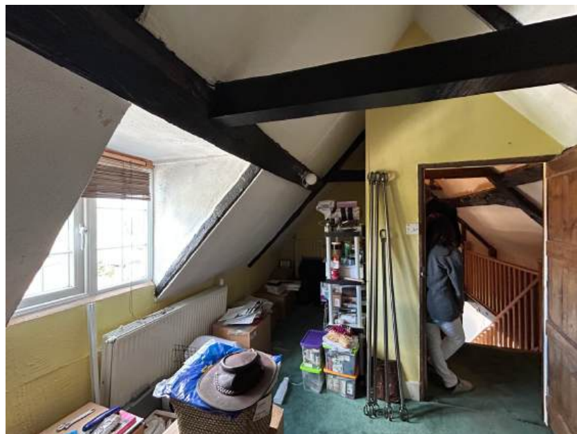
Fig 26-View of the 2 nd Floor attic room.
