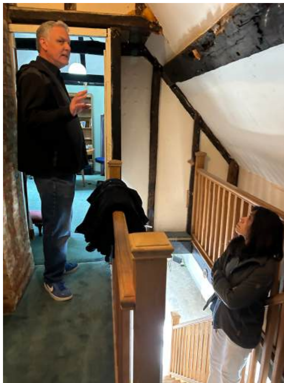
Fig 28-View of the stair landing with some planted-on original studwork moved from a different location.
