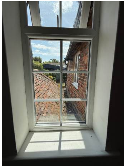
Fig 29-View of the kitchen extension roof
