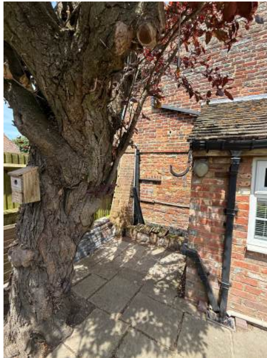
Fig 12– View of the blocked-up window
