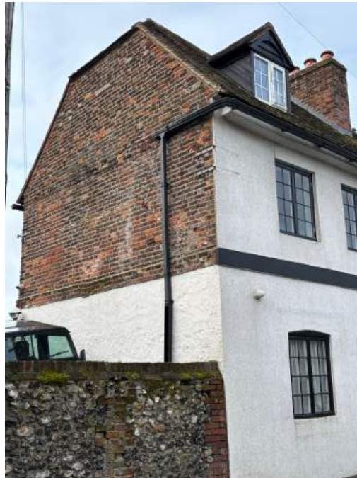
Fig 31-View of the flank elevation from the street.
