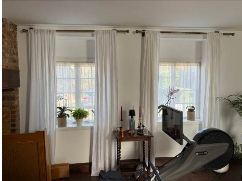
Fig 05 - View of the altered openings housing the 19 th C casement windows.
