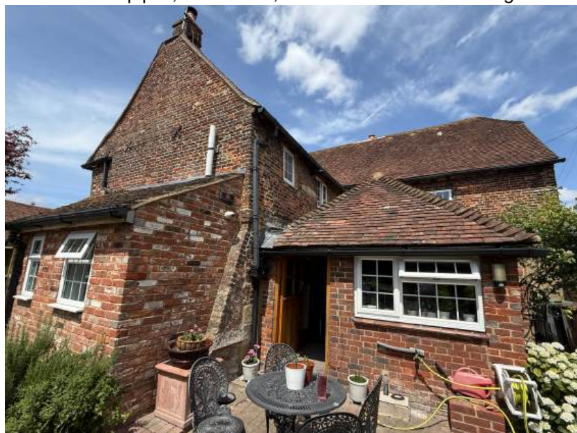
Fig 30-View of the rear of the house/drainage goods
