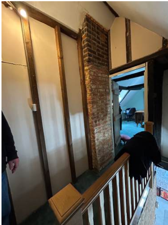
Fig 27-View of the 2 nd Floor stair landing, with planted-on modern studs.
