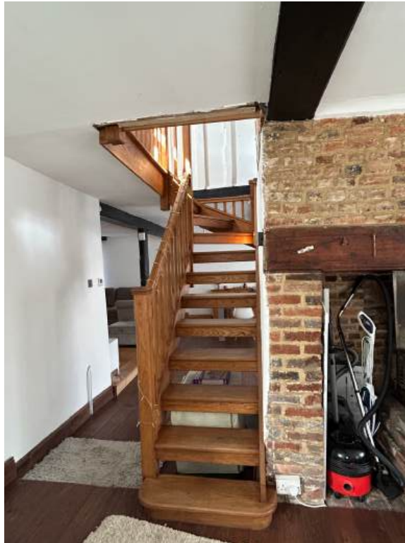
Fig 15 – View of the modern timber staircase inserted on the line of the removed original stud wall.
