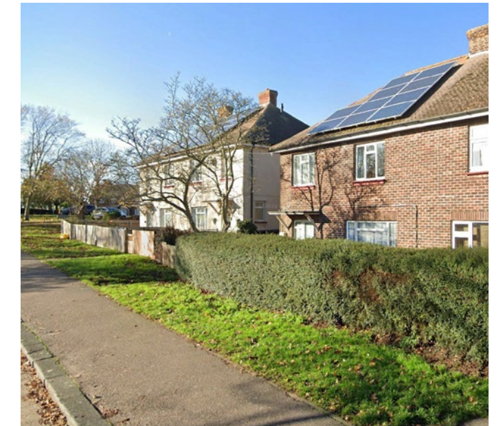
2 - SOLAR PANELS ON ROOFS
