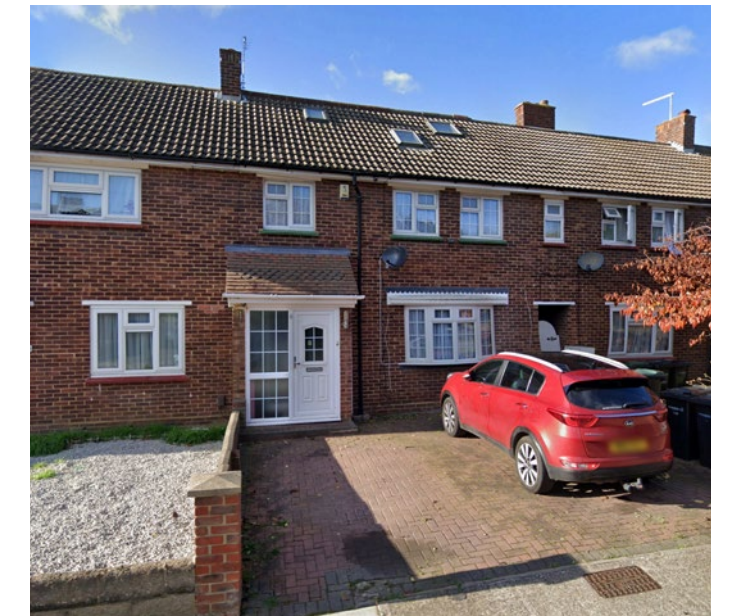
4 - ROW OF TERRACE HOUSING ALONG TENSING AVENUE
