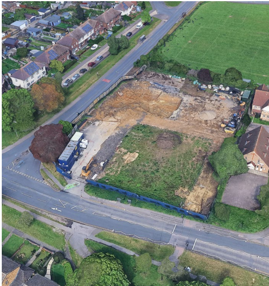
01 - GOOGLE EARTH AERIAL OF CONSTRUCTION SITE
