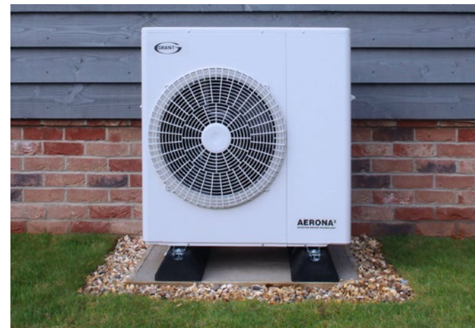
AIR SOURCE HEAT PUMPS
