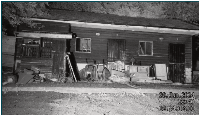
Photograph 1. NVA view of survey position S2
