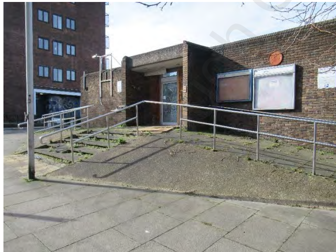
Plate 6. View of former pedestrian access off Windmill Street
