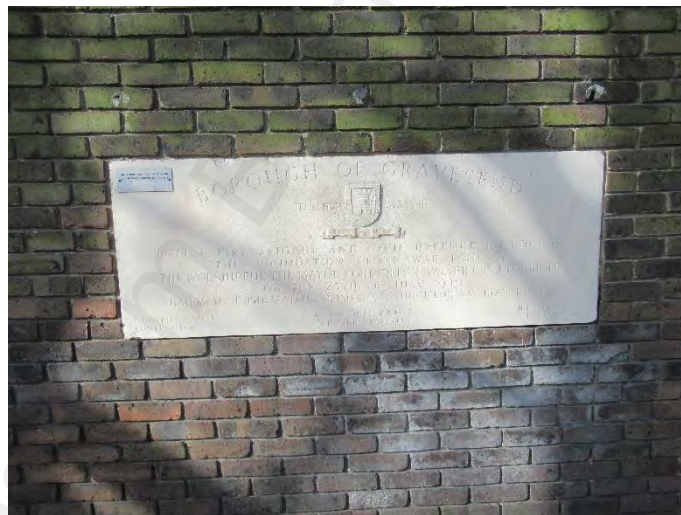
Plate 8. Foundation stone in the east boundary wall
