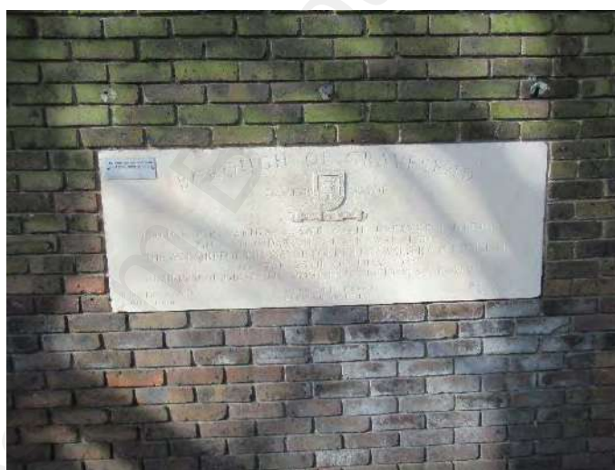
Plate 8. Foundation stone in the east boundary wall
