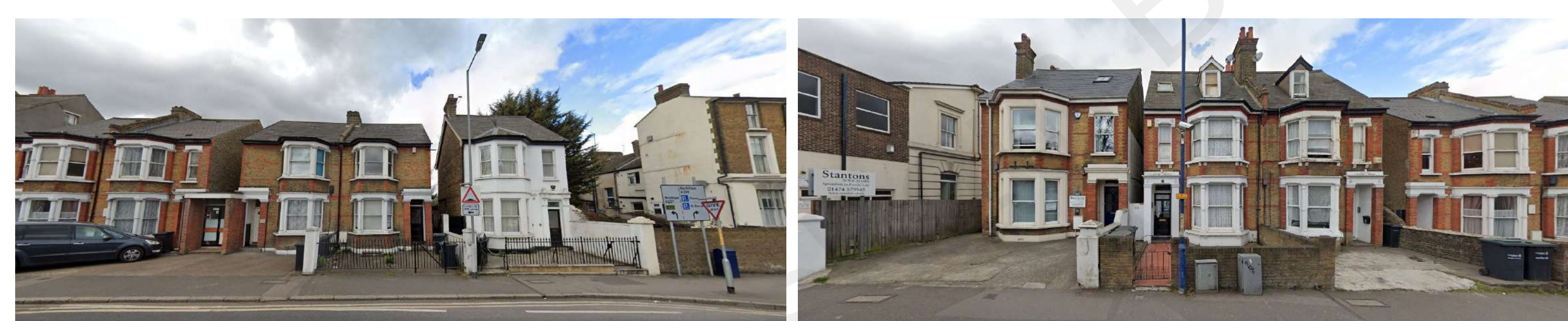
Wrotham Road Frontage
