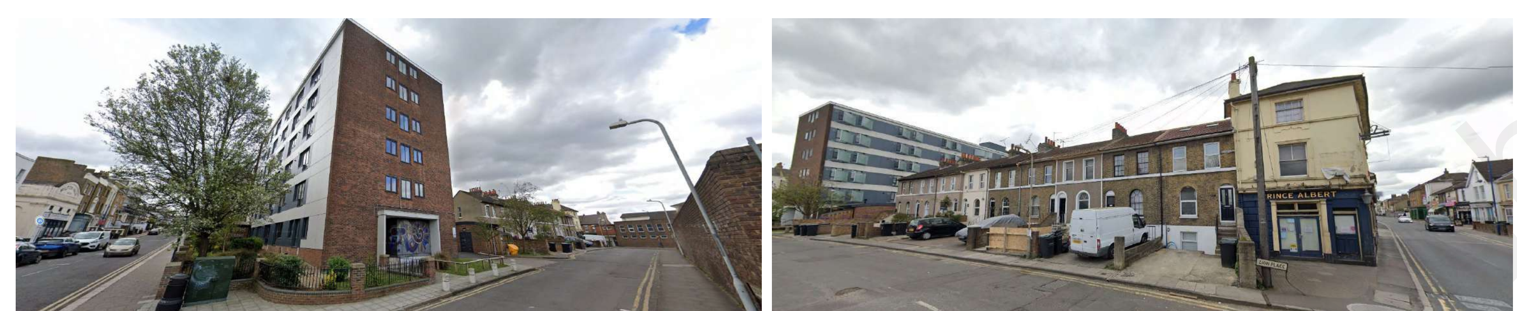
Zion Place Frontage
